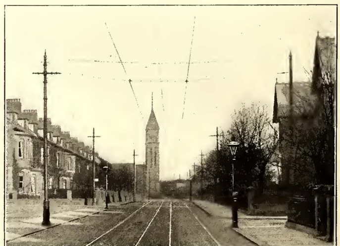
SPAN WIRE CONSTRUCTION ON OSBORNE ROAD
