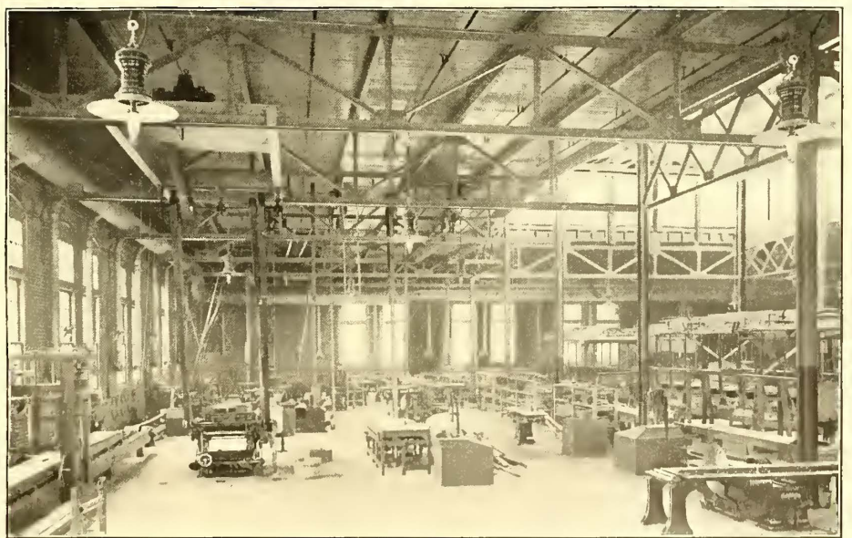
BLACKSMITH AND WOODWORKING SHOPS
