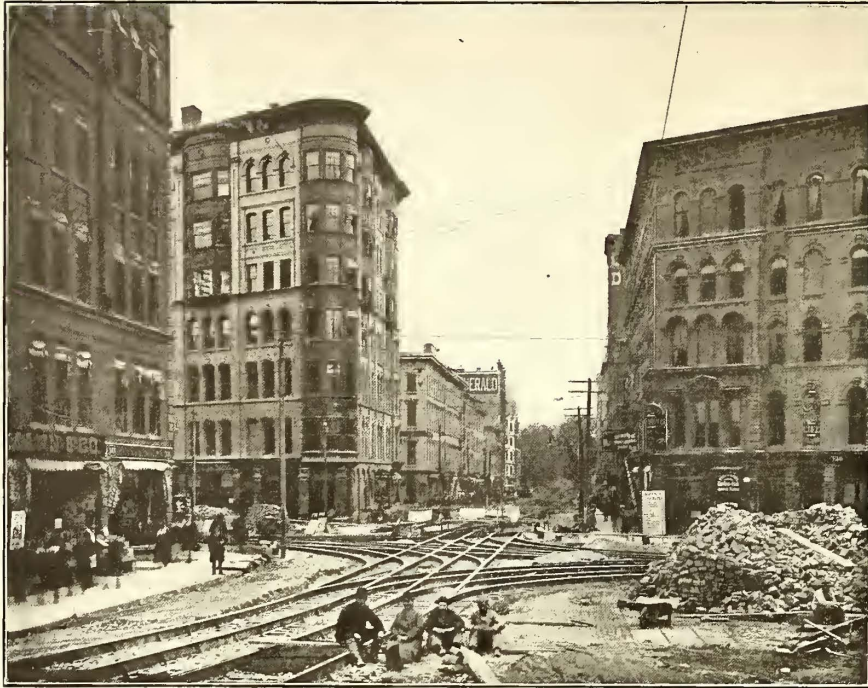
LAYING A HANDSOME PIECE OF SPECIAL WORK
