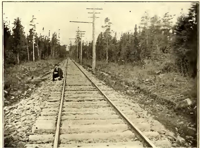
TRACK CONSTRUCTION THROUGH RECLAIMED SWAMP
