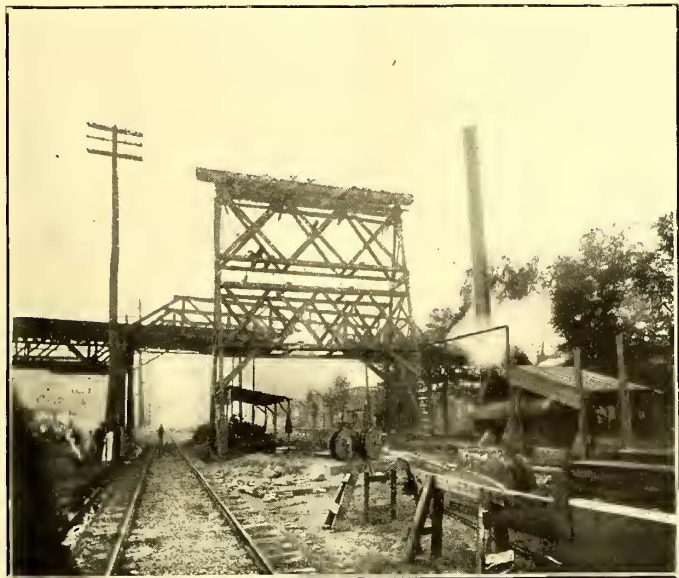
STRUCTURE AT END OF CABLEWAY
