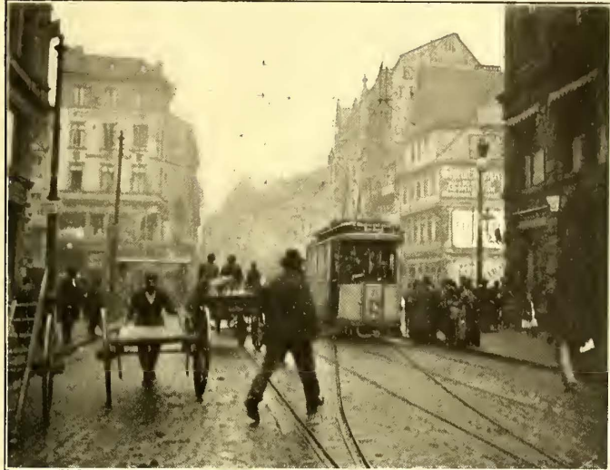
OVERHEAD GUARD WIRE CONSTRUCTION IN FRANKFORT
