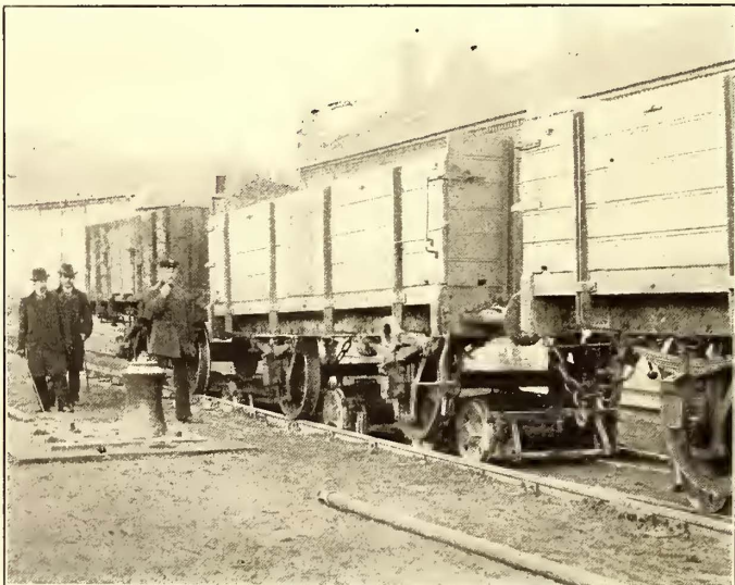
TRUCK USED FOR HAULING STANDARD GAGE STEAM CARS ON A NARROW GAGE ELECTRIC LINE, MEISSNERSTRASSENBAHN
