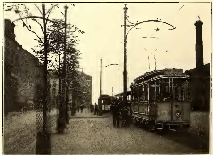
OVERHEAD CONSTRUCTION IN FRANKFORT, SHOWING TELEPHONE GUARD WIRES
