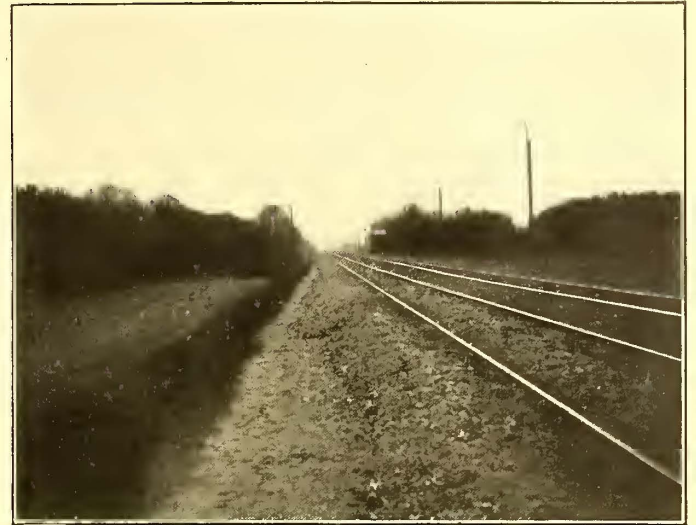
TRACK CONSTRUCTION ON ZOSSEN LINE
