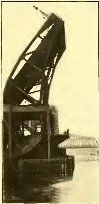
SCHERZER BRIDGE, OPEN
