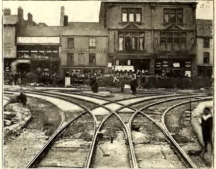
STREETS BEFORE PAVING, SHOWING HANDSOME SPECIAL WORK
