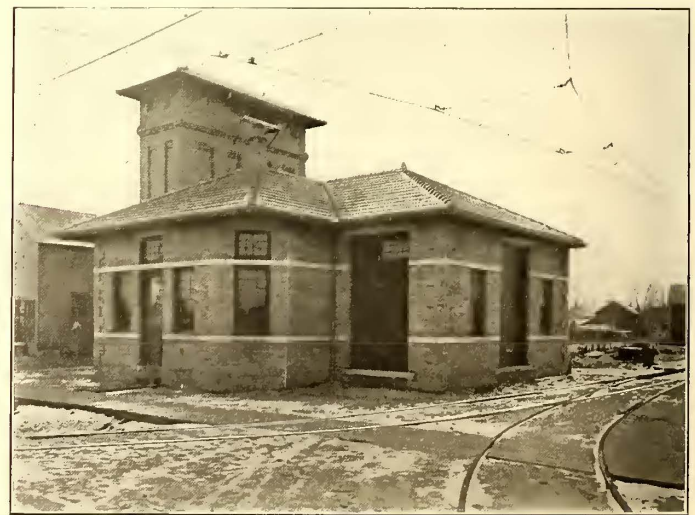
COOPERSVILLE SUB-STATION, SHOWING OVERHEAD CONSTRUCTION
