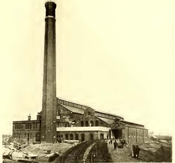
THE POWER STATION
