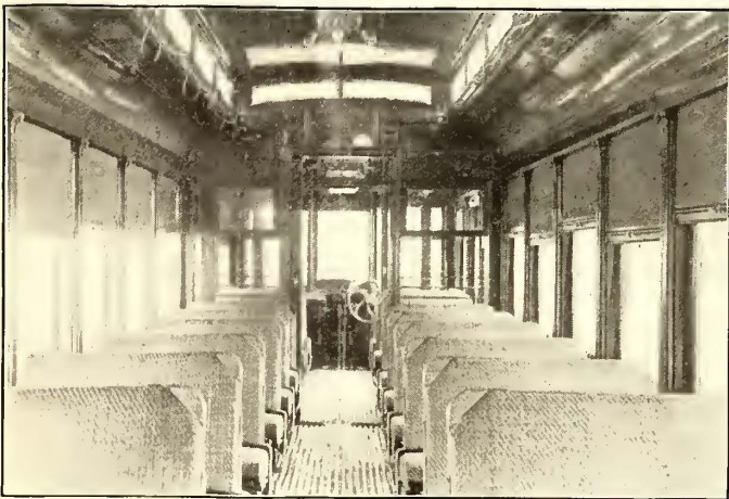
INTERIOR OF SUBURBAN CAR
