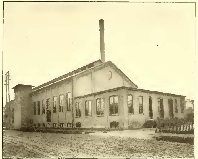
EXTERIOR OF POWER HOUSE
