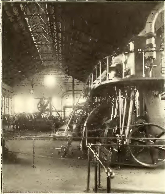
ONE OF THE LARGER ENGINES
