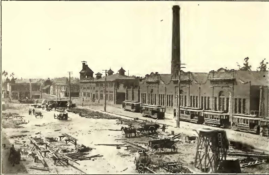
POWER STATION, SHOWING SITE OF NEW EXTENSION
