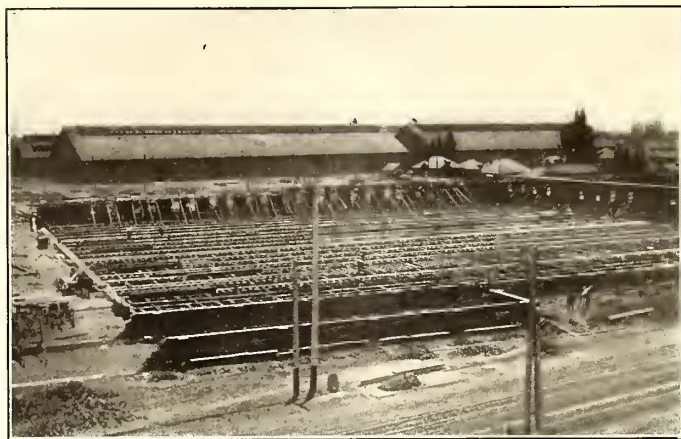
NEW CAR HOUSE UNDER CONSTRUCTION
