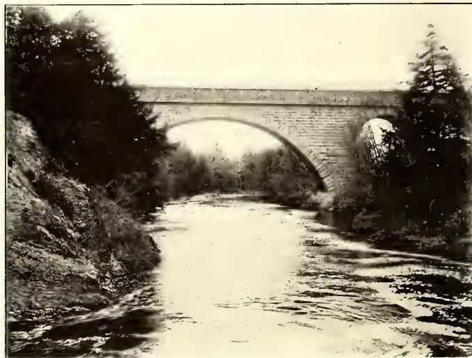
BRIDGE AT NEWTON
