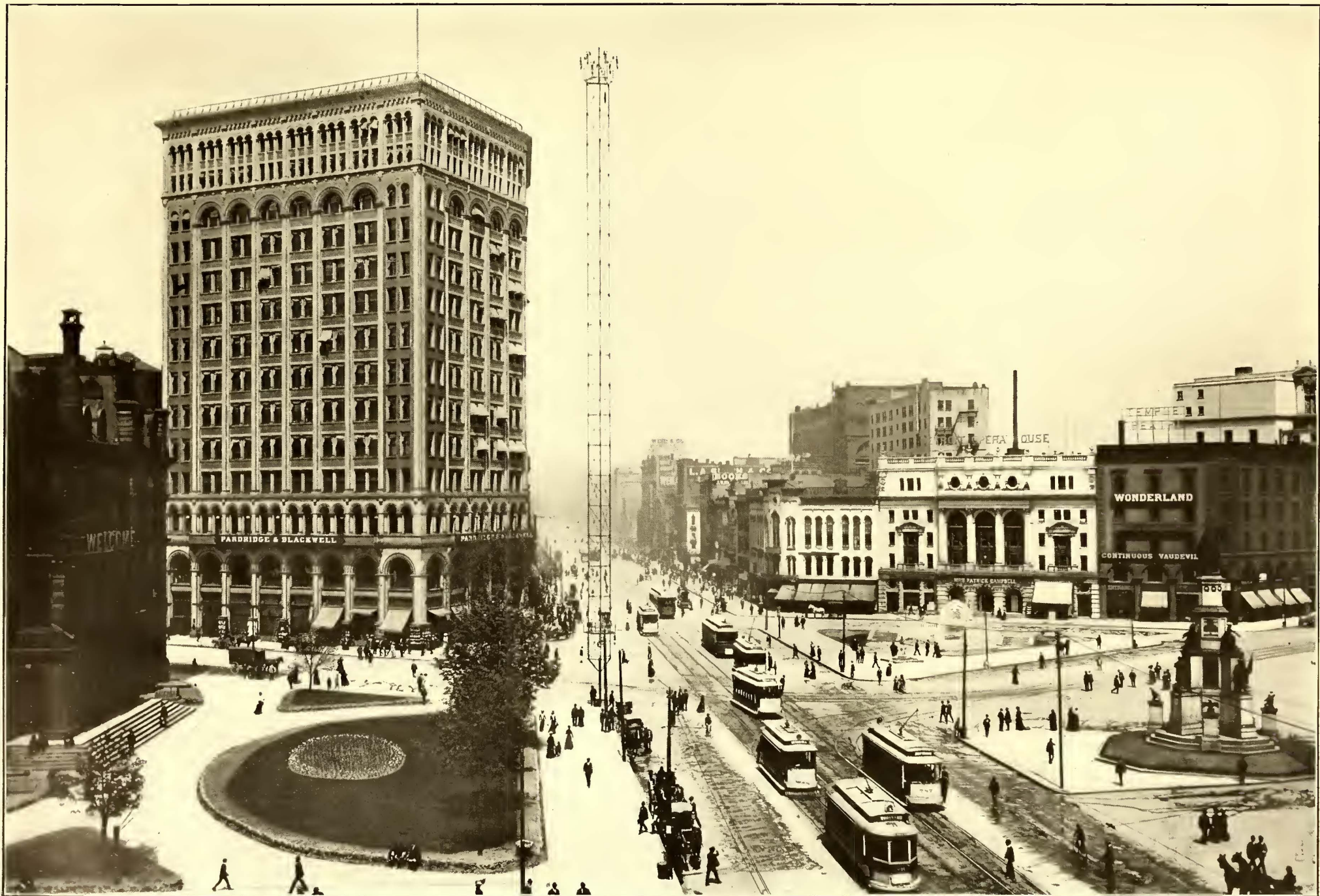
VIEW LOOKING UP WOODWARD AVENUE FROM THE CAMPUS MARTIUS, DETROIT
