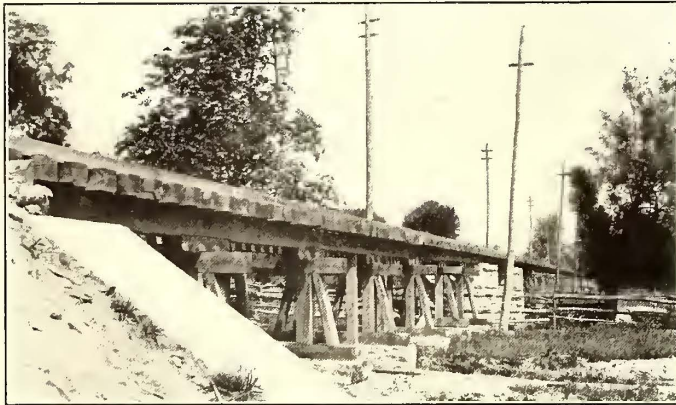
TRESTLEWORK NEAR READING
