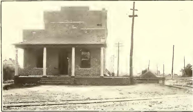
SUB-STATION, WAITING ROOM AND FREIGHT DEPOT, AT OXFORD
