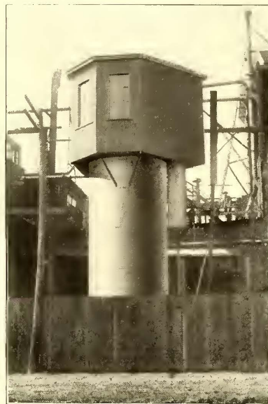
KENNICOTT WATER SOFTENING PLANT — TOP CLOSED
