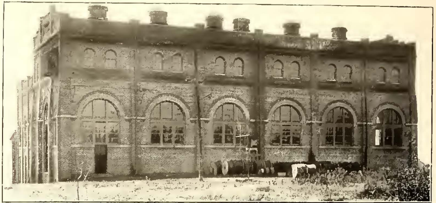
EXTERIOR OF STATION AT NEW BALTIMORE
