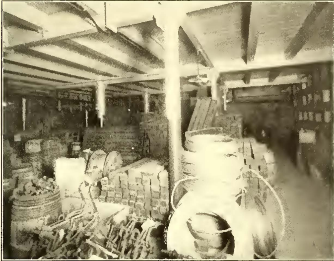
BASEMENT STOREROOM FOR WIRE AND HEAVY MATERIAL
