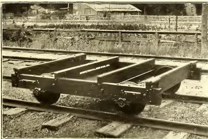
TRACK LAYING CARS
