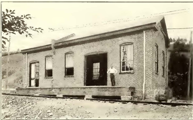
SUB-STATION NO. 2 AT SHANESVILLE
