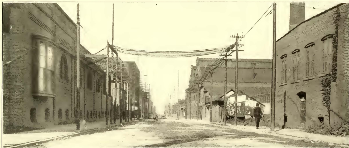
GENERATOR LEADS BETWEEN STATIONS A AND B
