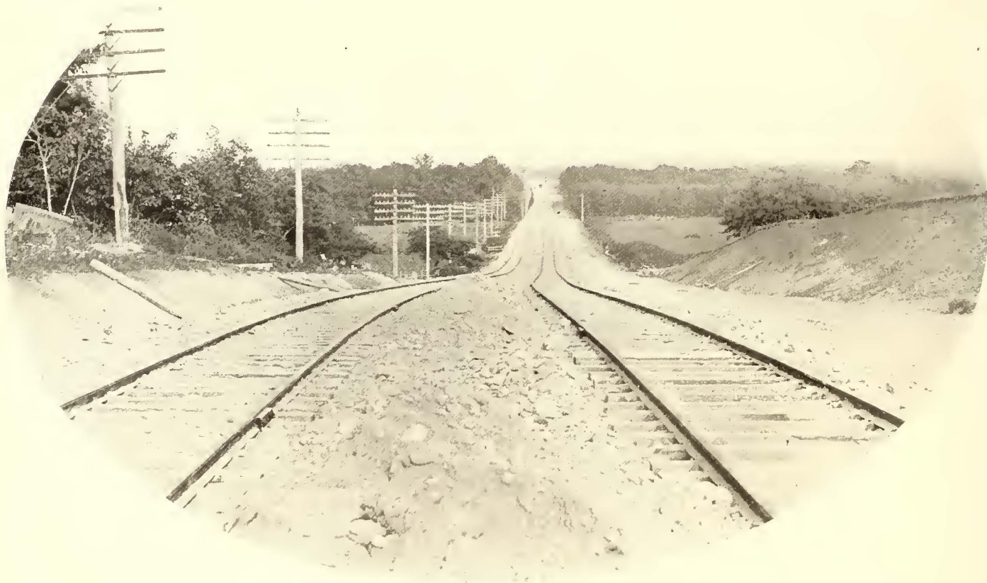
FRAMINGHAM BOULEVARD, LOOKING TOWARD BOSTON, WITH 20-FT. CARRIAGE WAY AT ONE SIDE
