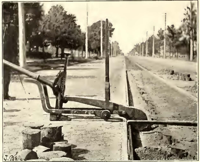
RAIL GROOVE SPREADER USED IN DETROIT
