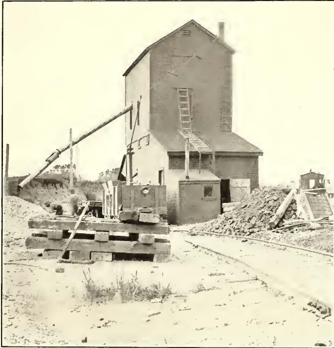
SAND DRYING PLANT AT A GRAVEL PIT
