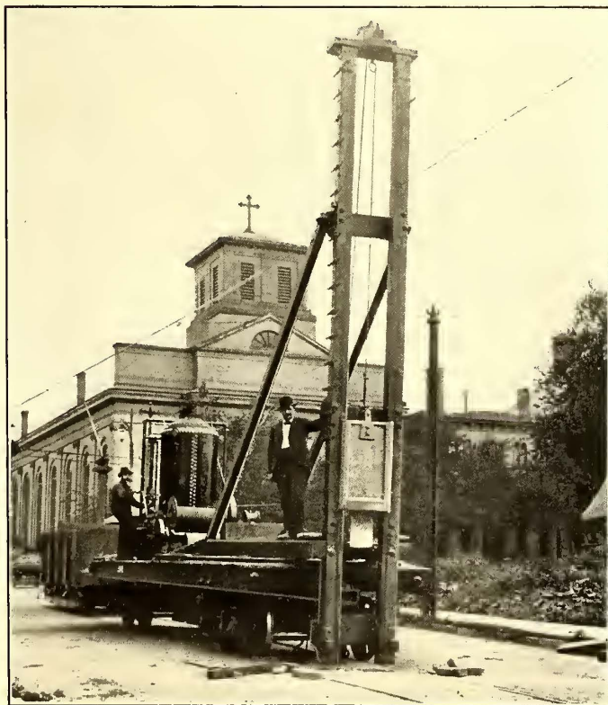
PILE DRIVER AS A CONCRETE BREAKER
