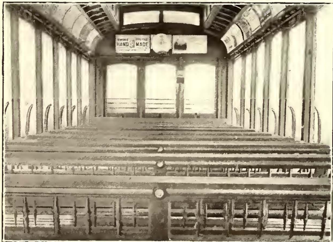
OPEN CAR SHOWING PUSH BUTTONS
