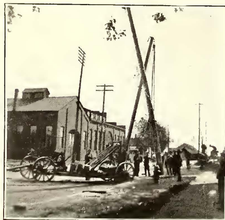
POLE PARTLY RAISED
