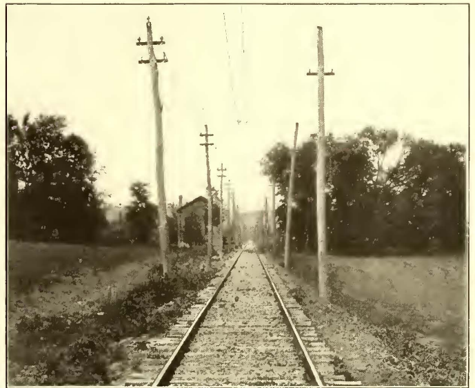
ROADBED AND OVERHEAD CONSTRUCTION
