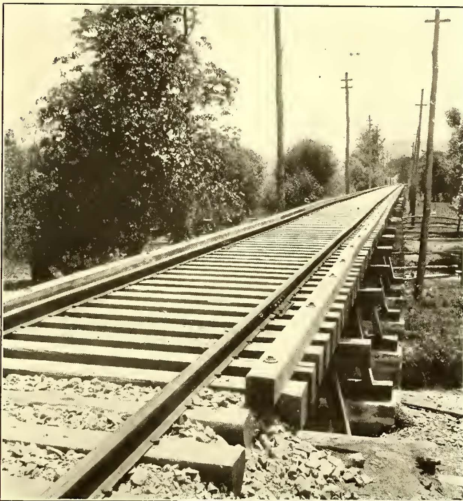
TRACK CONSTRUCTION AND BRIDGE WORK
