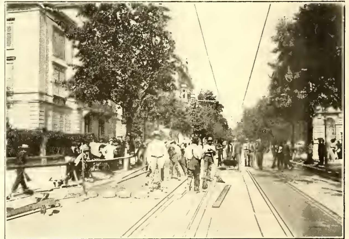
LAYING ASPHALT PAVING
