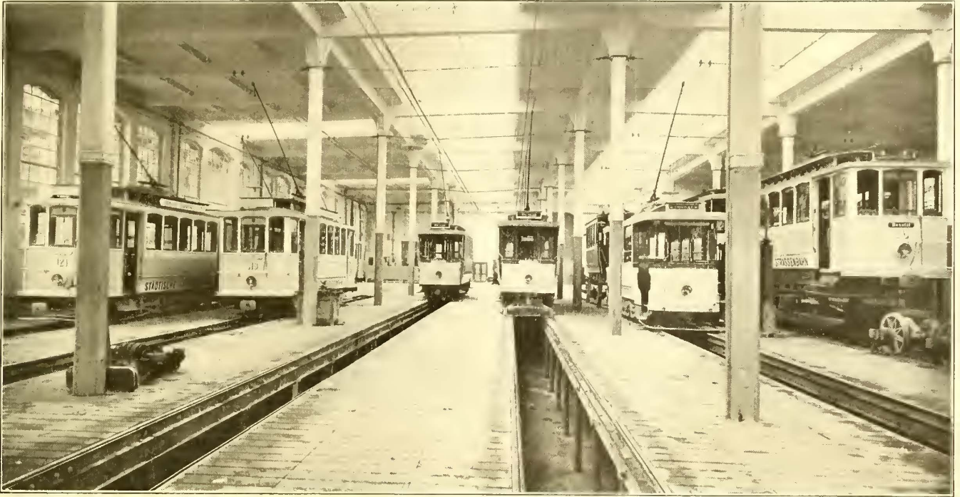
INTERIOR OF CAR HOUSE ON SEEFELDSTRASSE
