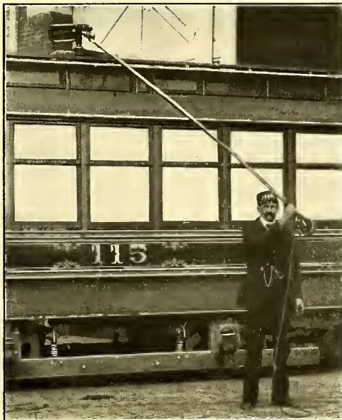
FIG. 10.—ADJUSTABLE TROLLEY POLE
