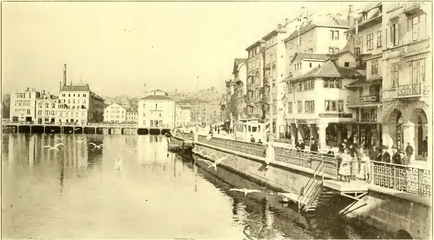
VIEW OF QUAY ALONG THE LIMMAT RIVER, ZURICH
