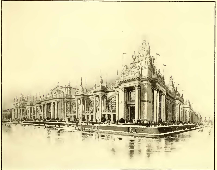
THE PALACE OF ELECTRICITY
