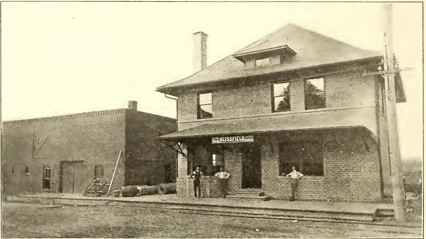
TYPICAL FREIGHT, EXPRESS AND PASSENGER STATION ON TOLEDO & WESTERN RAILWAY
