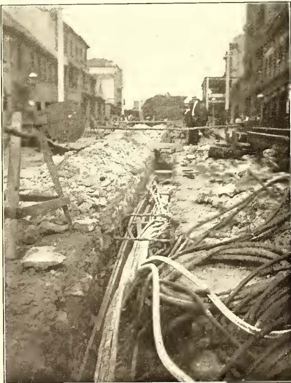
LAYING HIGH TENSION CABLES IN SYDNEY
