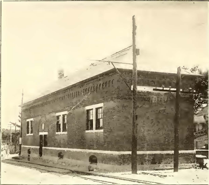
ONE OF THE SUB-STATIONS.
