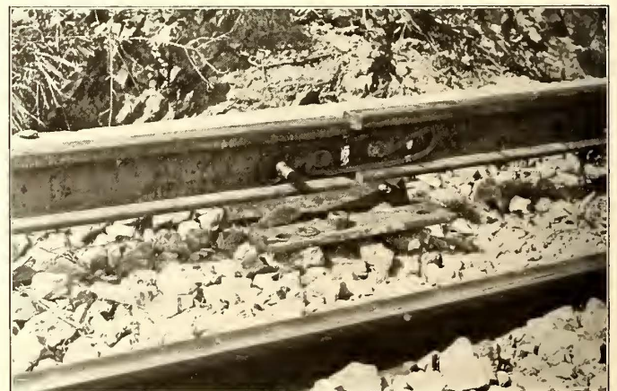
THIRD-RAIL EXPANSION JOINT, WITH PLATE REMOVED
