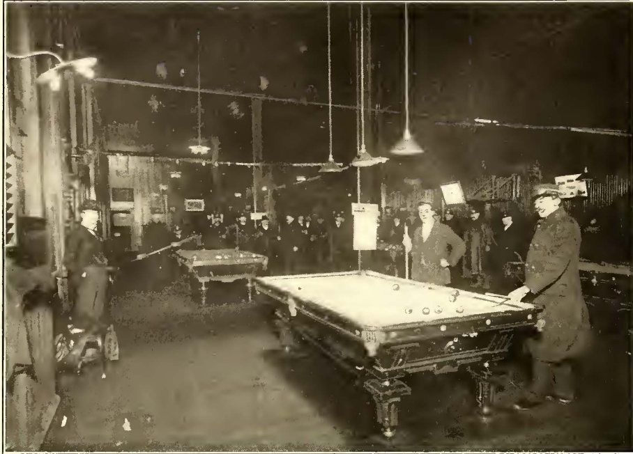
BILLIARD ROOM IN CROSTOWN DEPOT
