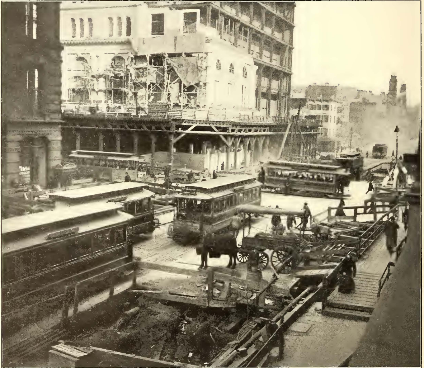
OBSTRUCTIONS AT TWENTY-THIRD STREET AND FOURTH AVENUE
