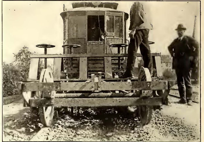
END VIEW, SHOWING PLOWS DOWN
