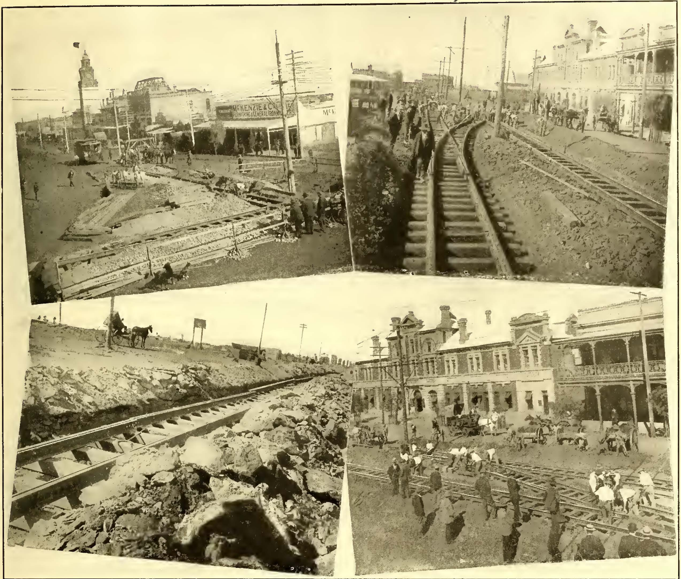
VIEWS SHOWING PORTIONS OF THE ROAD IN COURSE OF CONSTRUCTION
