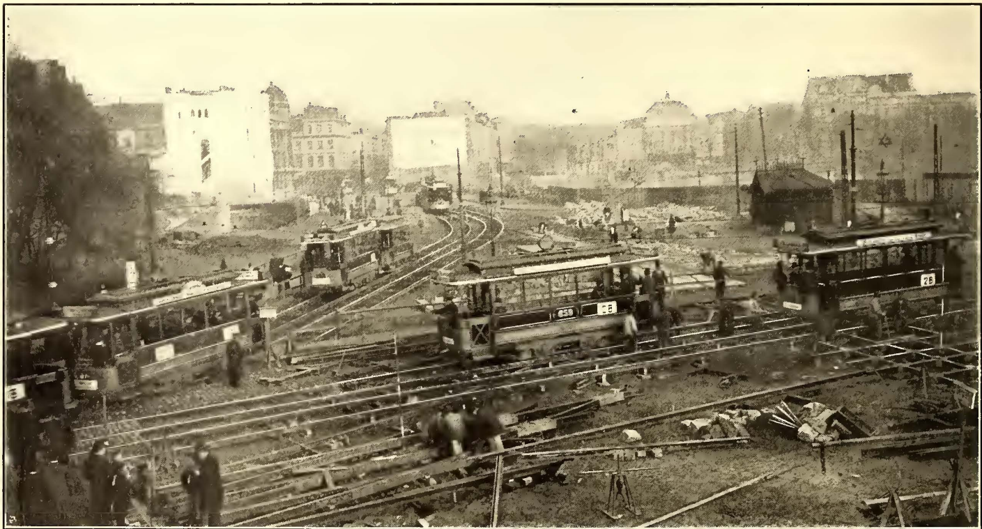
INTERESTING TRACK WORK IN HAMBURG
