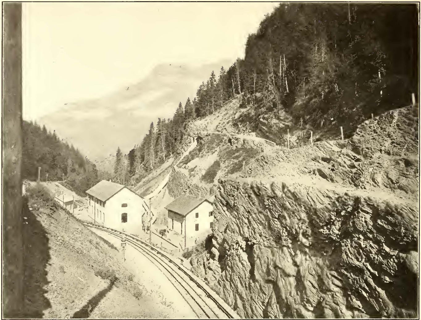
HYDRAULIC POWER STATION AT SERVOZ
