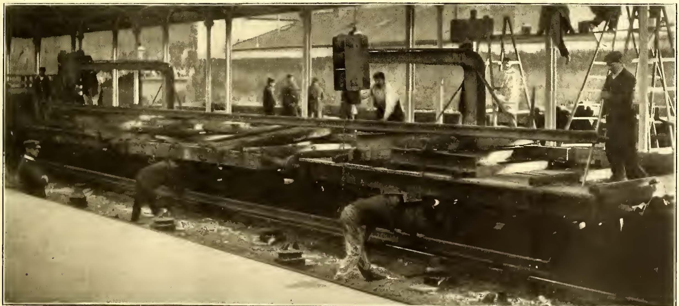
METHOD OF LAYING THIRD RAIL
