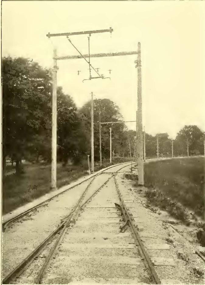
THREE-PHASE HIGH-TENSION OVERHEAD CROSSING, BUDA-PEST EXPERIMENTAL RAILWAY
