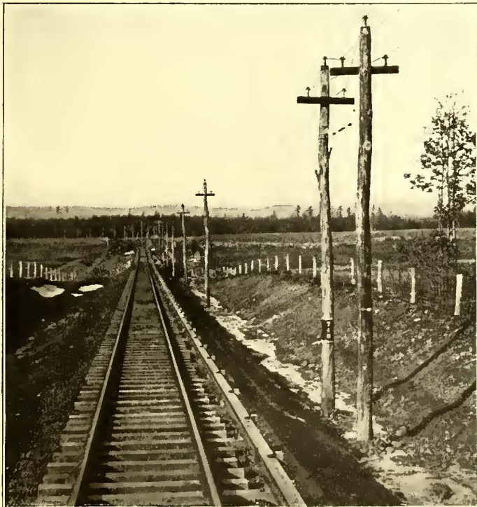
TRANSPPOSITION POLES IN HIGH-TENSION LINE
