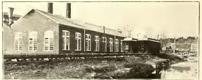
POWER HOUSE AT ST. JOHNS
