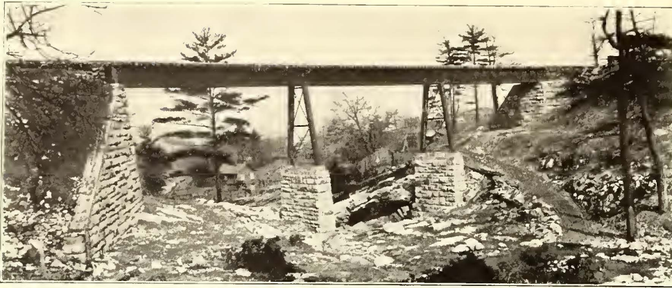
BRIDGE WORK OVER SOLOMON'S GAP
