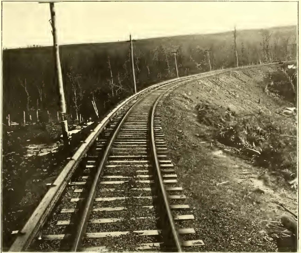
POLE LINE AND TRACK CONSTRUCTION OVER LONG FILL AND CURVE
