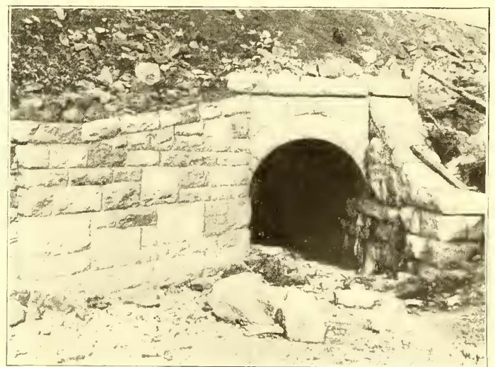
CULVERT AT SUGAR NOTCH RUN
