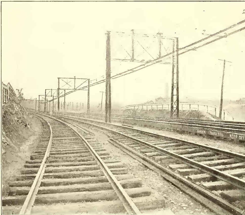
VIEW SHOWING PRESENT THIRD RAIL AND OLD OVERHEAD CONSTRUCTION
