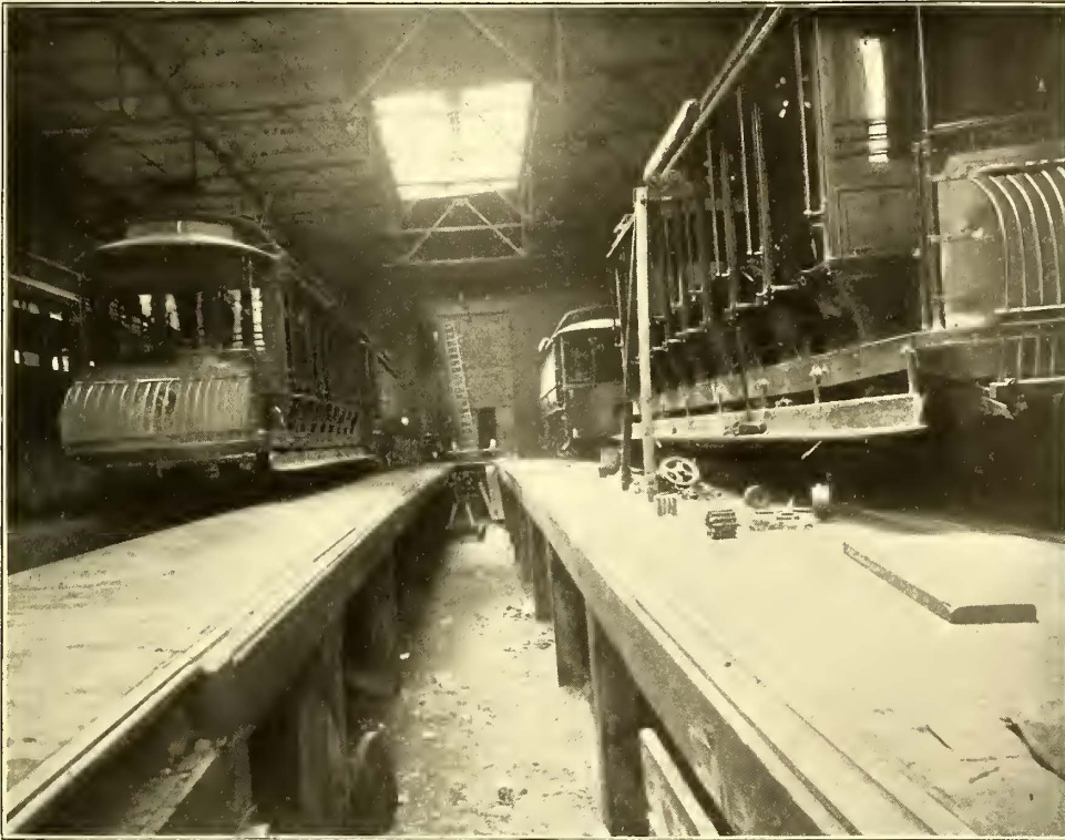
FIG. 5.—VIEW OF LARGE CAR SHEDS, WITH INCOMPLETE CUT-OFF, UNPROTECTED ROOF TRUSSES, UNSATISFACTORY PITS, AND WITHOUT STANDARD DIVISION WALLS
