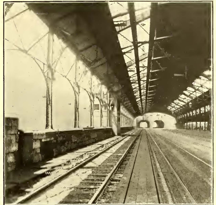
VIEW IN MT. ROYAL STATION, SHOWING PROTECTED THIRD RAIL
