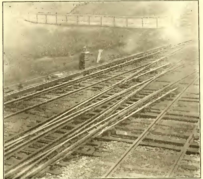
VIEW OF SLIP SWITCHES AT HUNTINGTON AVENUE, SHOWING MOVABLE THIRD RAIL
