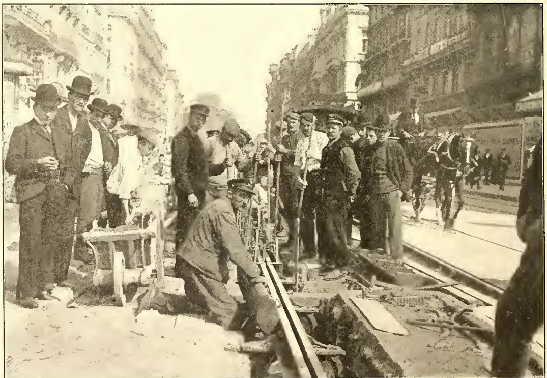
INSERTING MOULDS IN TRENCH
