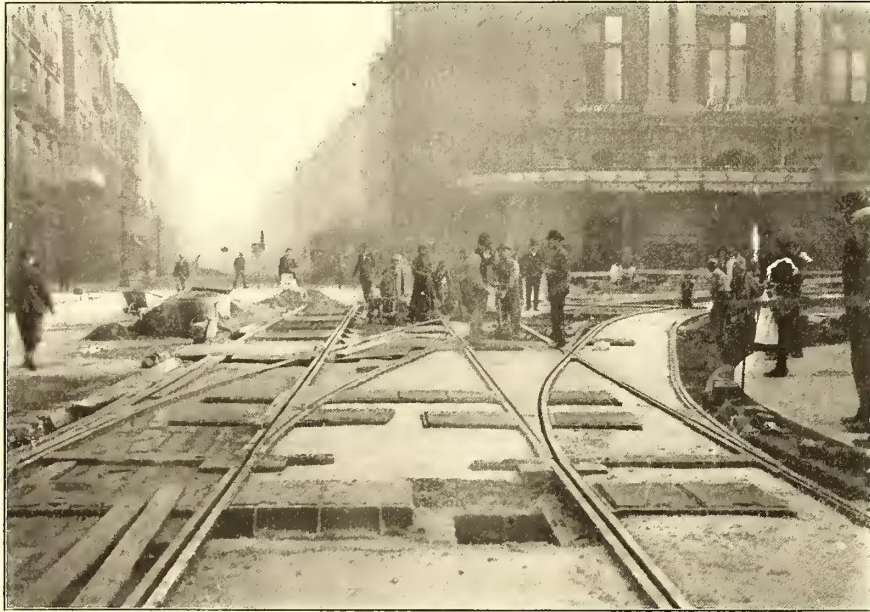
VIEW OF PARTIALLY COMPLETED WORK
