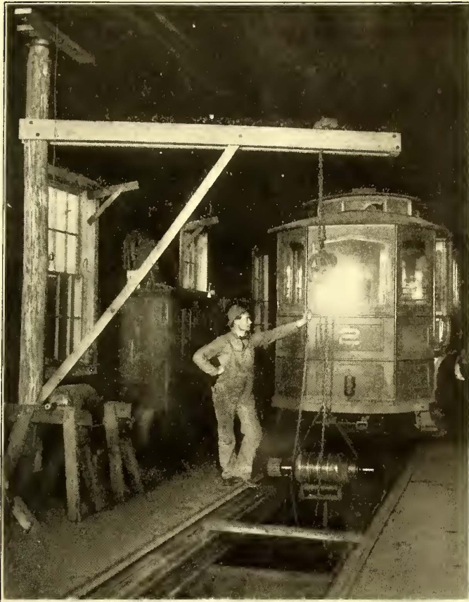
HANDLING ARMATURES IN CAR HOUSE
