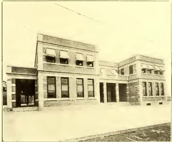
FRONT OF SCRANTON PASSENGER STATION
