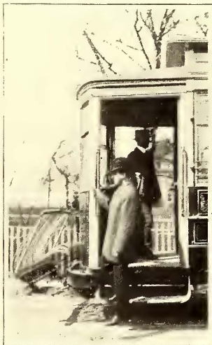
INCORRECT--Very Dangerous! GETTING OFF IN OPPOSITE DIRECTION CAR TRAVELS.
