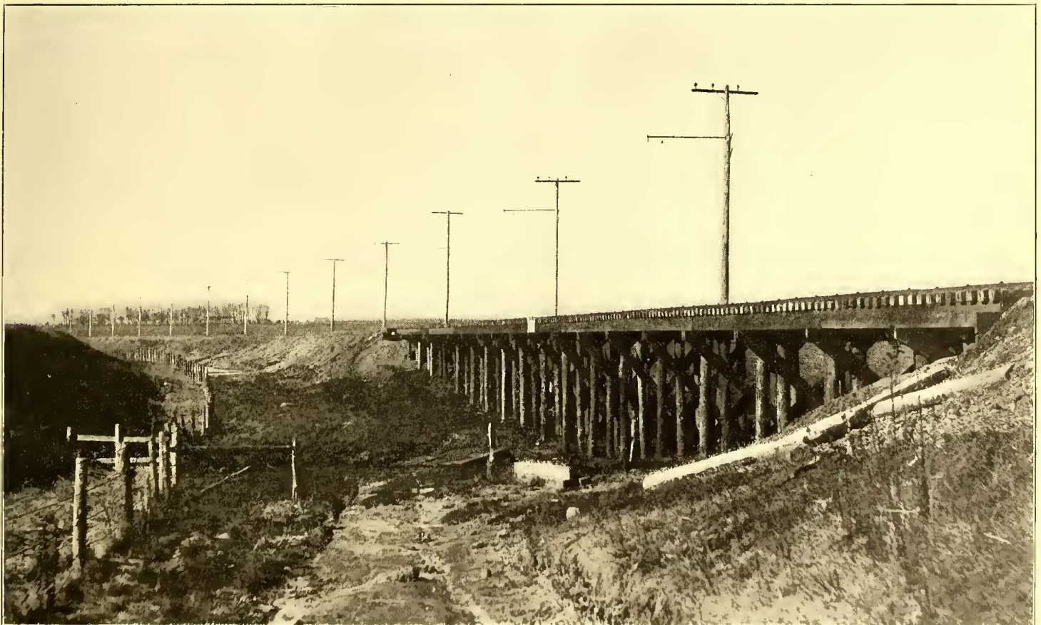
TRESTLE AND FILL
