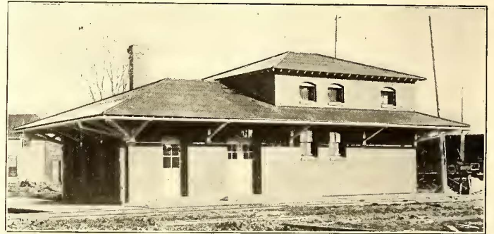
SUB-STATION AT MITCHELLVILLE
