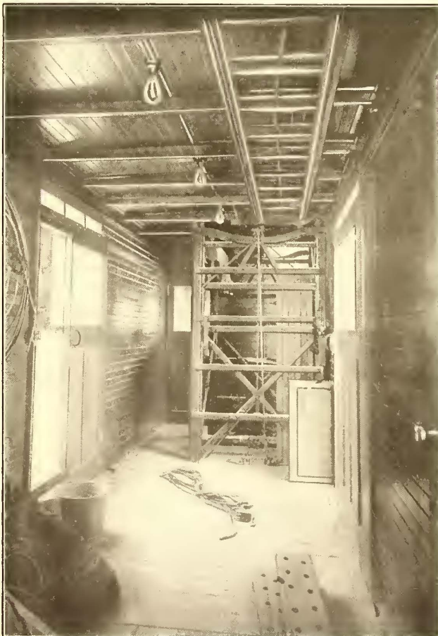
FIG. 7.—INTERIOR OF EMERGENCY CAR
