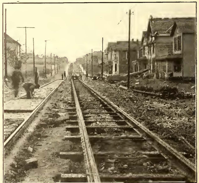
FIG. 4.—VIEW ON SUMMIT STREET, SHOWING SPACING OF TIES AND TIE BARS
