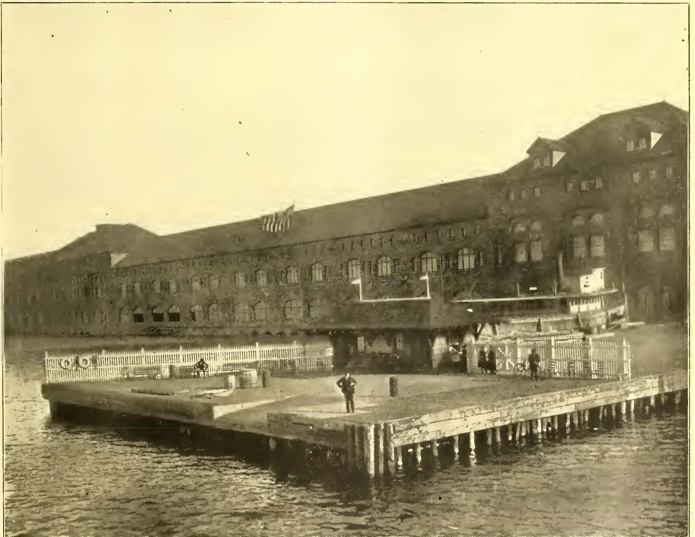
POWER HOUSE AND RAILWAY TERMINAL DOCK ON AMERICAN SIDE
