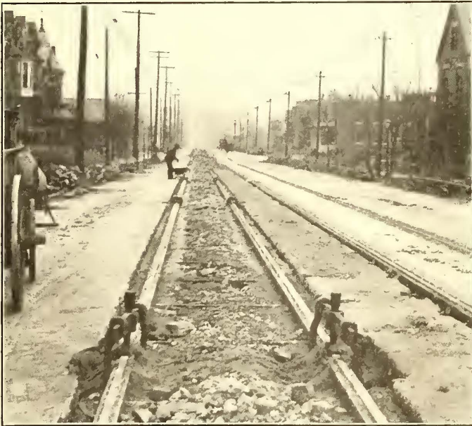
FIG. 1.—MOULDS SET READY FOR WELDING
