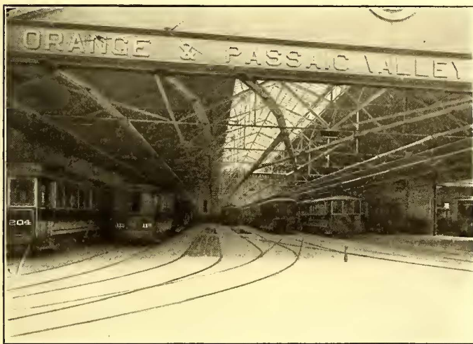
FIG. 2.—INTERIOR OF CAR HOUSE
