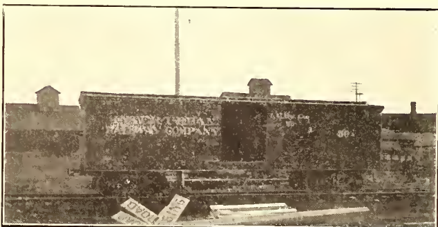
FIG. 3.—BOX FREIGHT CAR USED AS TRAILER IN DES MOINES
