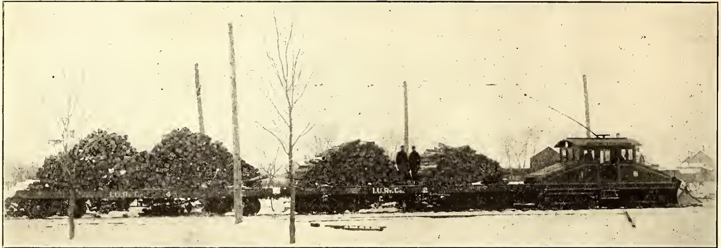
FIG. 5.— ELECTRIC FREIGHT TRAIN IN DES MOINES
