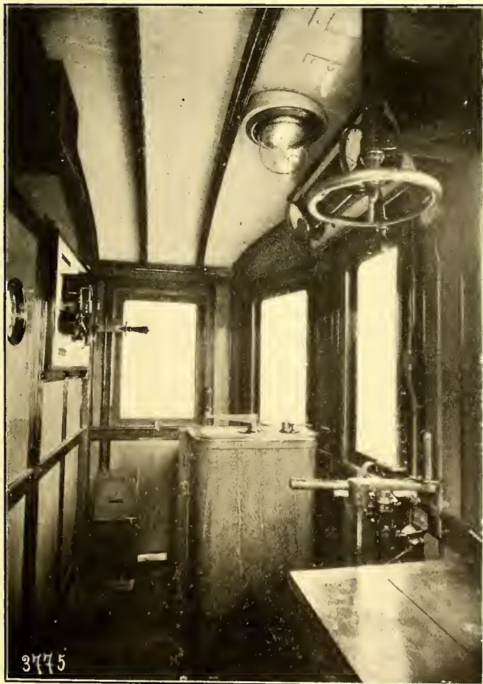
INTERIOR OF MOTORMAN'S COMPARTMENT, SHOWING CONTROLLING APPARATUS
