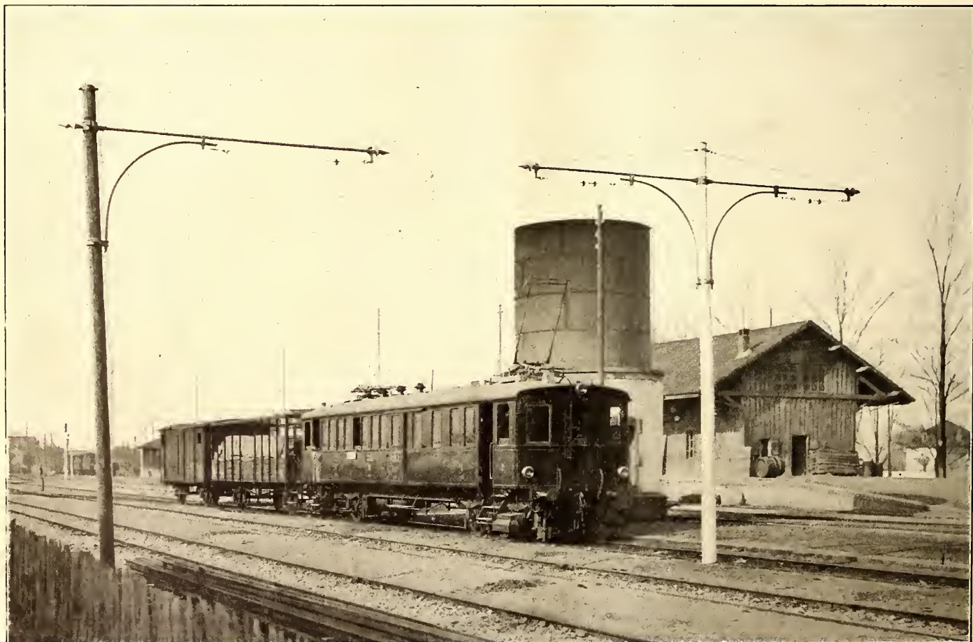
ELECTRIC FREIGHT TRAIN IN STATION AT MORAT
