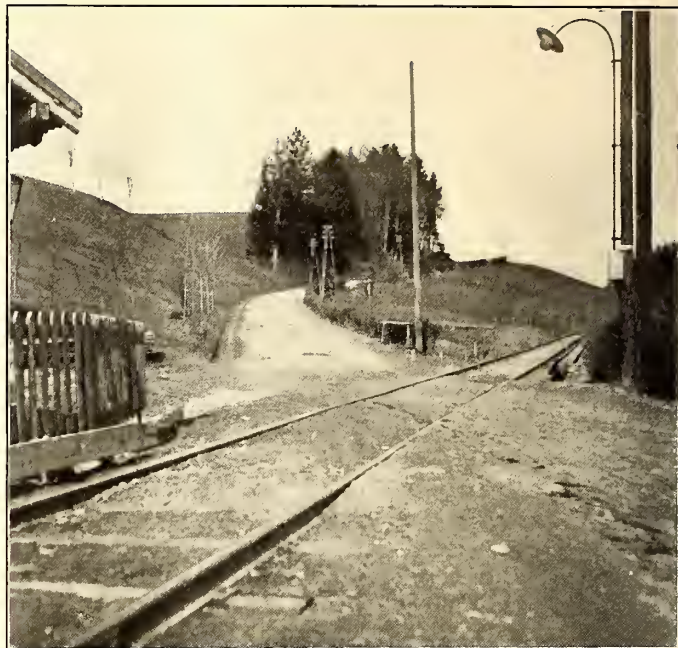
GRADE CROSSING WHERE THIRD RAIL IS CHANGED FROM ONE SIDE TO THE OTHER TO SECURE A SHORT BREAK
