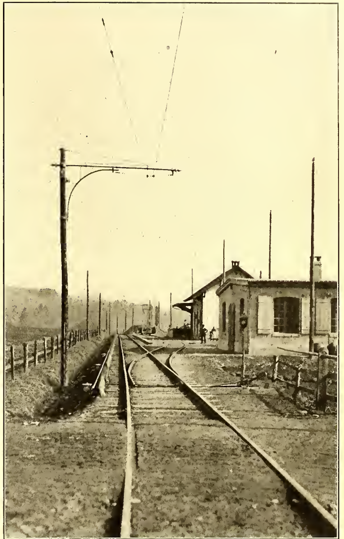
SUB-STATION AND PASSENGER STATION AT PENSIER, SHOWING A POINT WHERE CHANGE IS MADE FROM THIRD RAIL TO OVERHEAD WIRE
