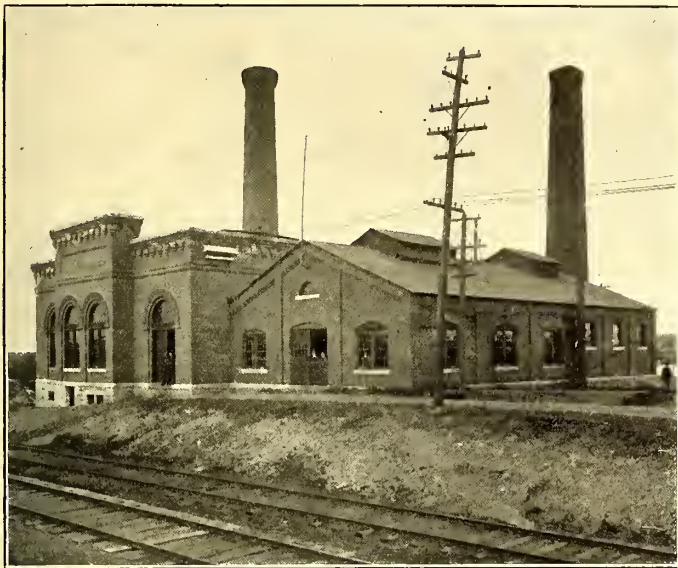
MAIN POWER HOUSE
