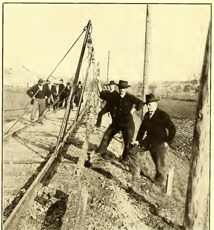
APPARATUS FOR SETTING THIRD RAIL IN POSITION
