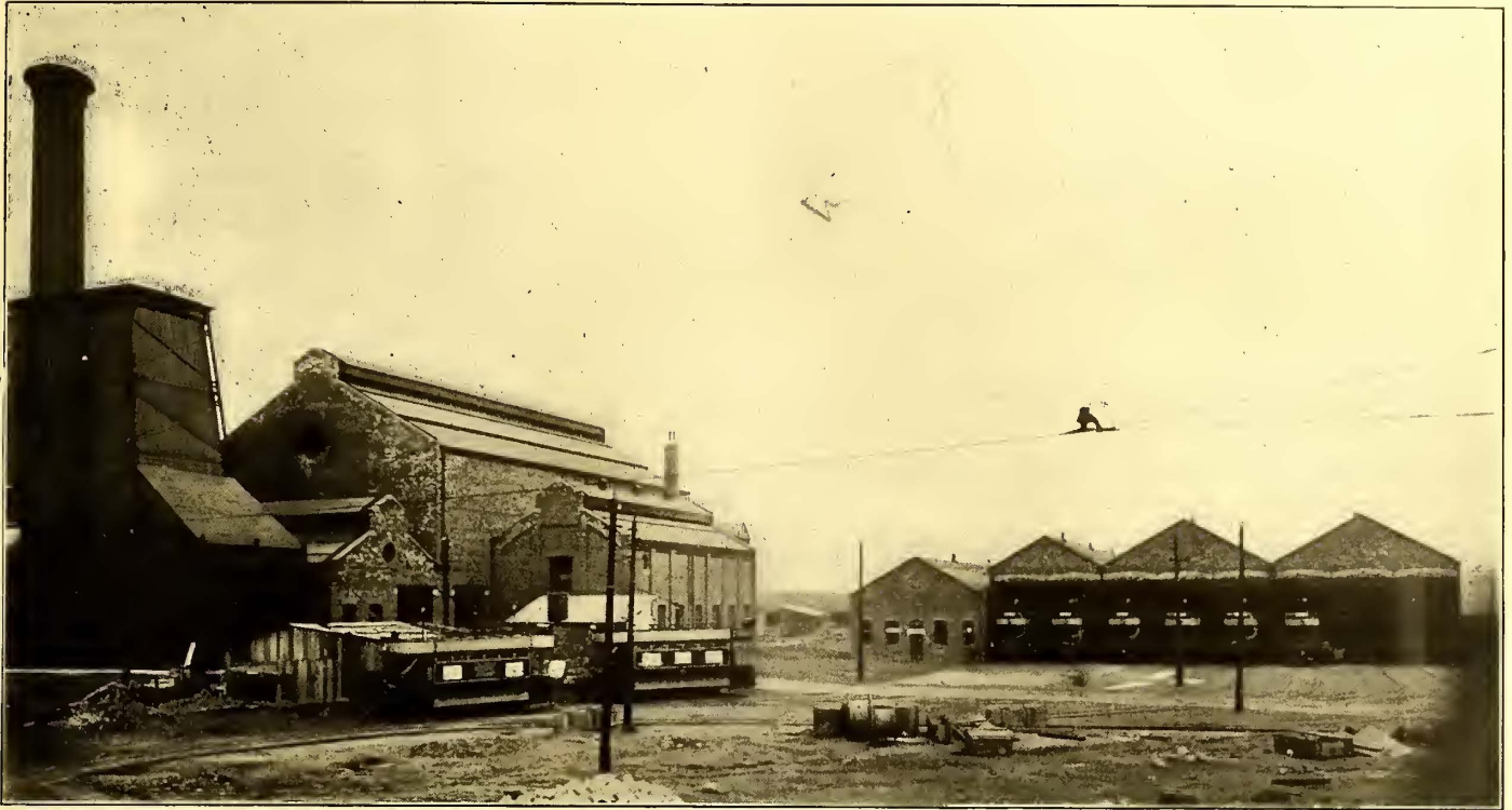
EXTERIOR OF POWER HOUSE AND CAR DEPOT AT ATHERTON
