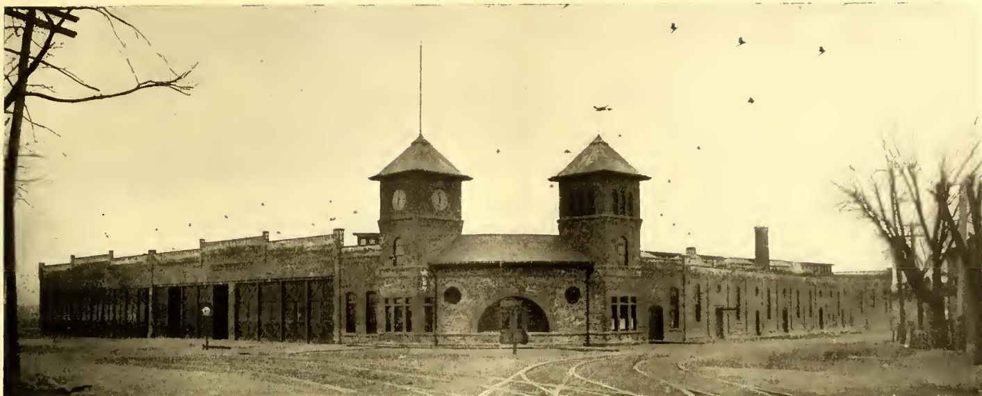
EXTERIOR OF CAR HOUSE AND REPAIR SHOPS AT WOODSIDE
