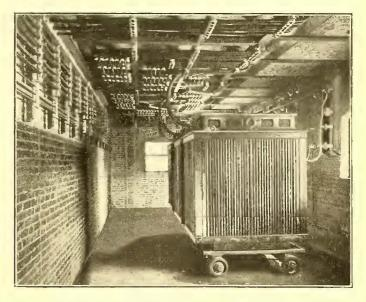
FIG. 7.-VIEW OF TRANSFORMER ROOM, DIRECTLY BELOW SWITCHBOARD IN AUBURN POWER HOUSE
