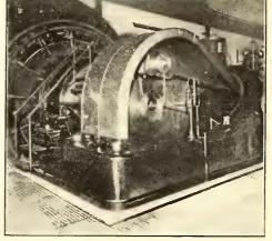
wheel housing placed around a 20-ft. fly-wheel on a Wetherill engine in the Mt. Vernon station of the Philadelphia Rapid Transit Company. This particular construction was adopted by the engineers of that company, because. owing to changes in the engines and generators at that station, it became necessary to mount
