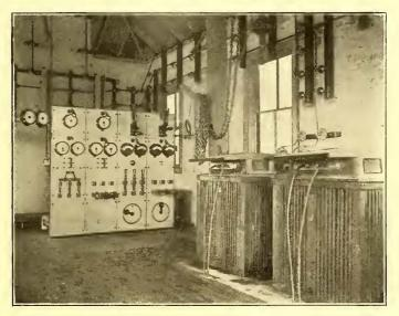
FIG. 9.--SWITCHBOARD AND TRANSFORMERS IN HOWLETT HILL SUB-STATION
