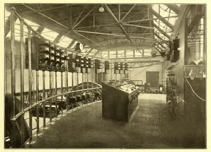
FIG. 5.—SWITCHBOARD GALLERY IN MAIN STATION, WITH DIRECT-CURRENT APPARATUS AT RIGHT, BENCHBOARD IN CENTER, AND ALTERNATING-CURRENT MEASURING INSTRUMENTS ON FRAMEWORK AT LEFT
