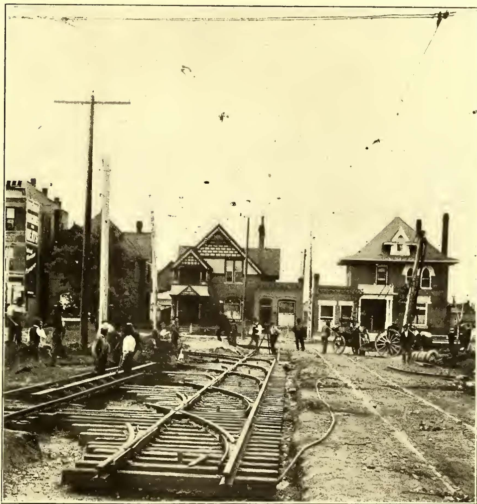
FIG. 28.—SPECIAL WORK FOR NEW CAR HOUSE; POLE RAISING EQUIPMENT
