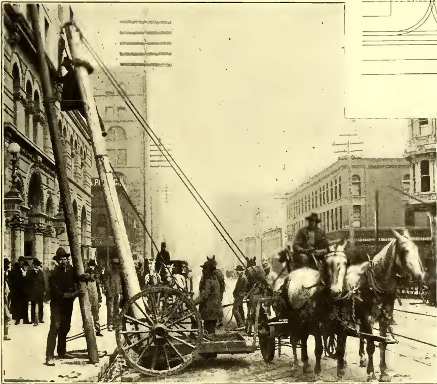
FIG. 23.—POLE SETTING WAGON
