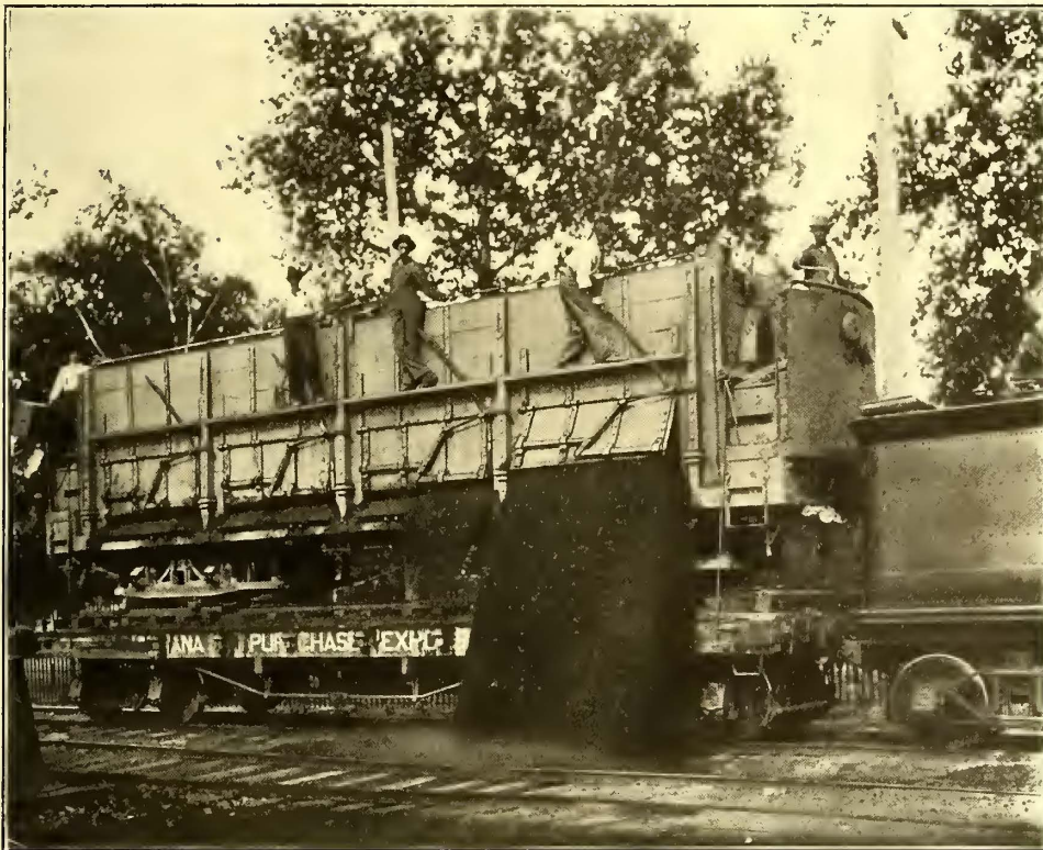
ELECTRIC DUMP-CAR MOUNTED ON FLAT-CAR AND DRAWN BY LOCOMOTIVE FOR DISTRIBUTING CINDERS IN ROADBED CONSTRUCTION
