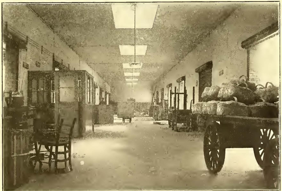
GENERAL INTERIOR VIEW
