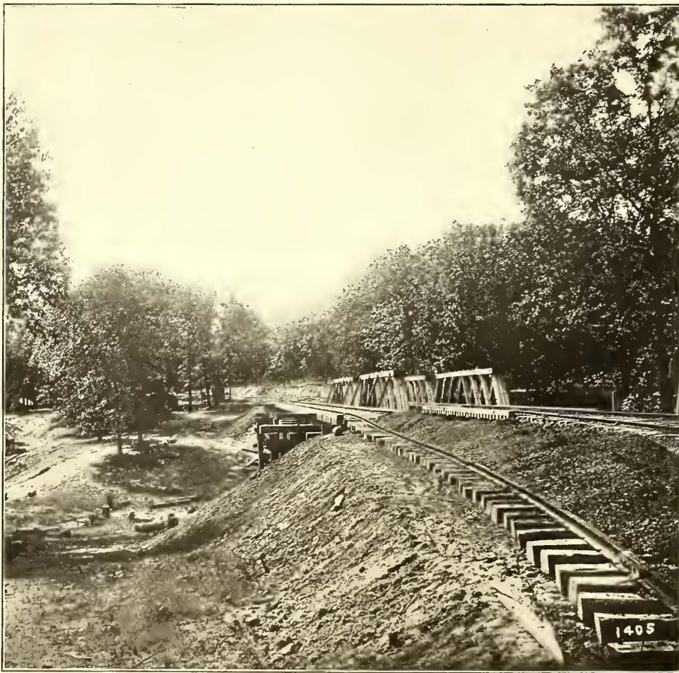
RAILWAY BRIDGE CROSSING RAVINE
