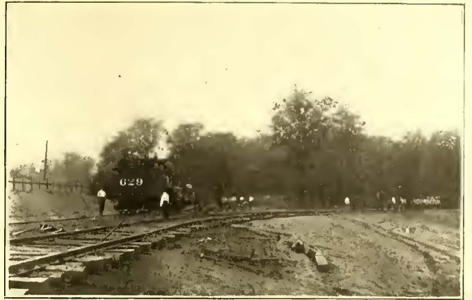
LAYING CONNECTION ON INTRAMURAL IN SOUTHERN PART OF GROUNDS
