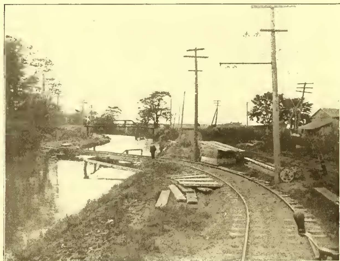
TIMBER DRAW-BRIDGE USED IN CONSTRUCTION
