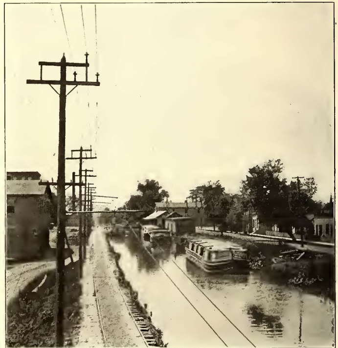
VIEW ALONG CANAL, SHOWING LINE AND TRACK.
