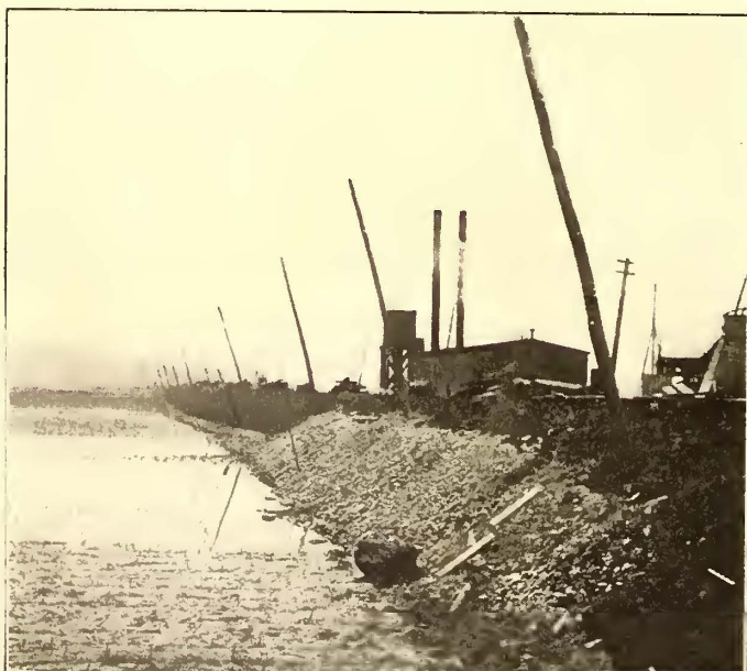
FILL, NEAR CINCINNATI, SHOWING RIP-RAP BEING PLACED ON IT
