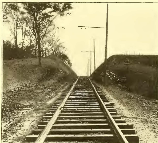
CUT 557 FT. LONG, 40 FT. DEEP, NEAR LEBANON (RAPID DIVISION)
