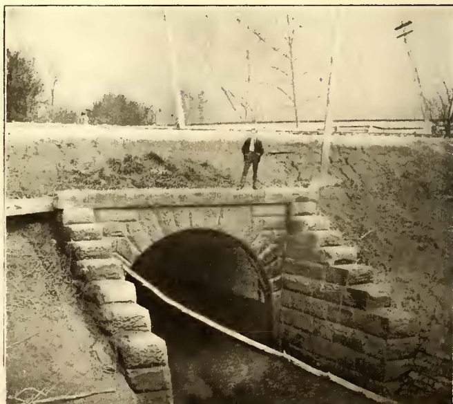
10-FT. BRICK, CONCRETE AND STONE ARCH CULVERT (SUBURBAN DIVISION)
