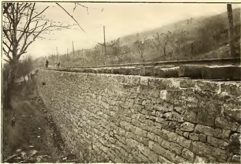
RETAINING WALL (CINCINNATI &amp; EASTERN DIVISION)
