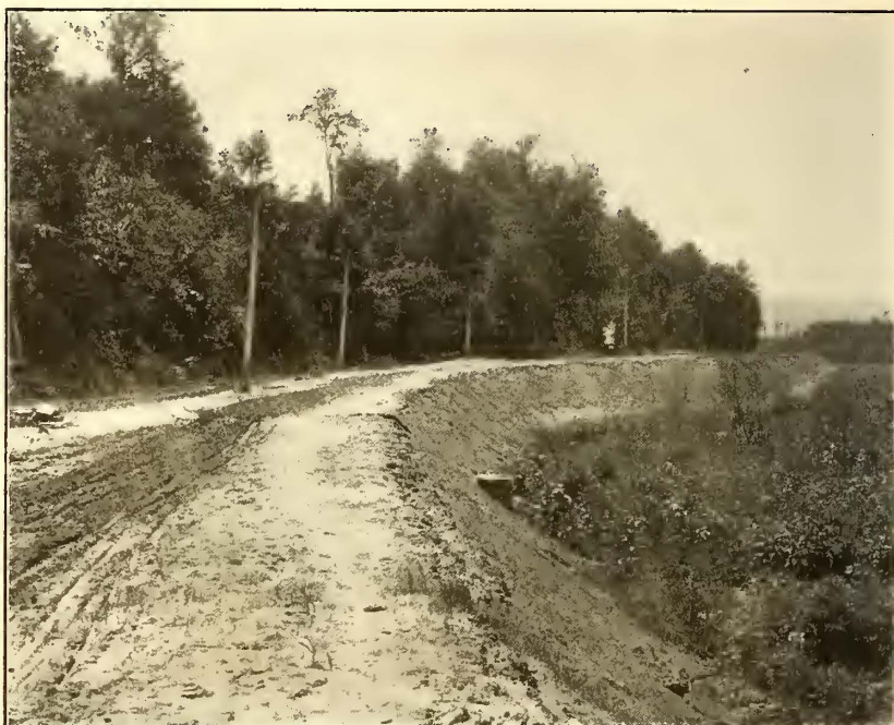
FILL THROUGH APPROACH NEAR NEW WATERWORKS (CINCINNATI & EASTERN DIVISION)
