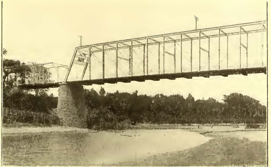
MIAMI RIVER BRIDGE (CINCINNATI & EASTERN DIVISION)
