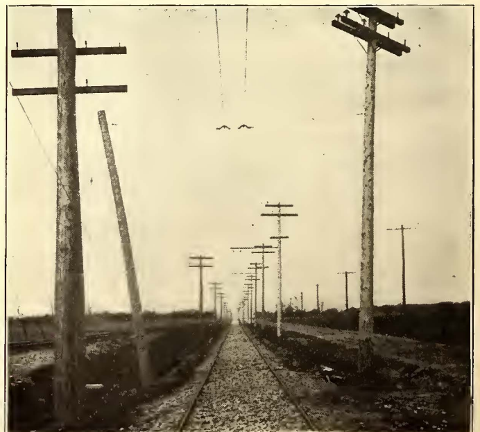
SINGLE-TRACK, SIDE-POLE BRACKET CONSTRUCTION
