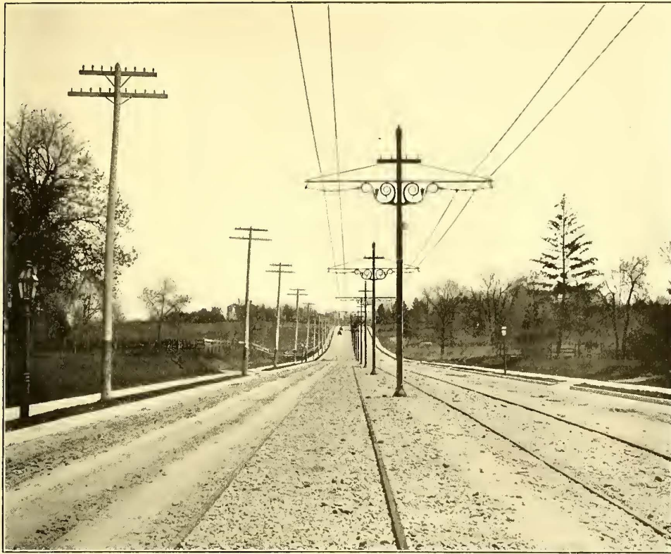
DOUBLE-TRACK, CENTER-POLE BRACKET CONSTRUCTION (RAPID RAILWAY DIVISION)
