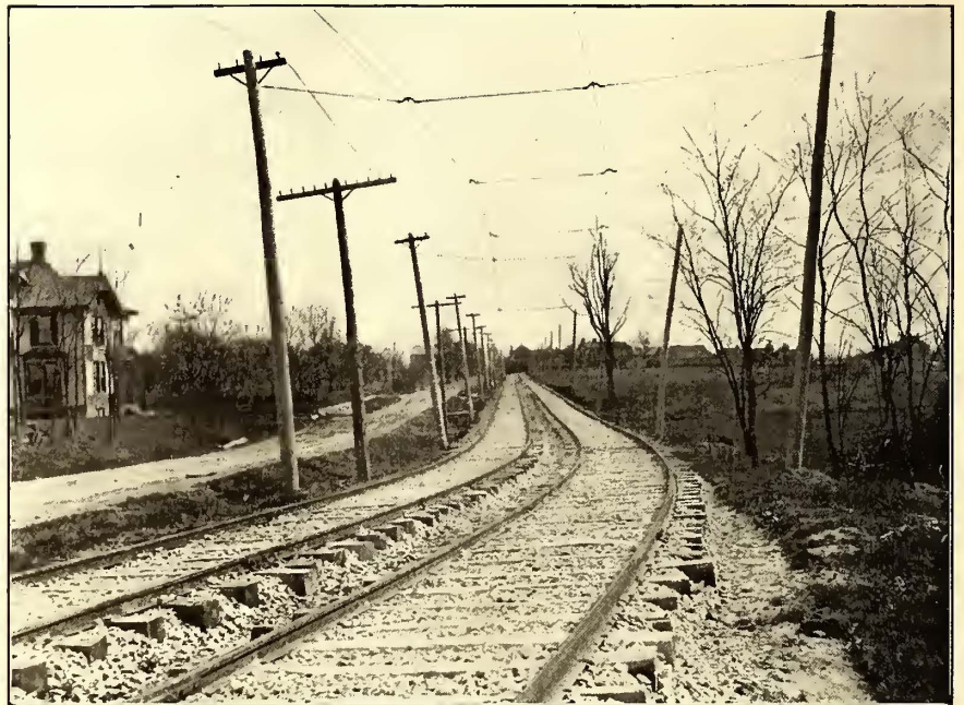
DOUBLE-TRACK SPAN CONSTRUCTION
