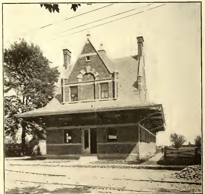
SUB-STATION AND DEPOT AT AMELIA, OHIO, SUBURBAN DIVISION (LIVING ROOM FOR ATTENDANT UPSTAIRS OVER GENERAL WAITING ROOM IN FRONT)
