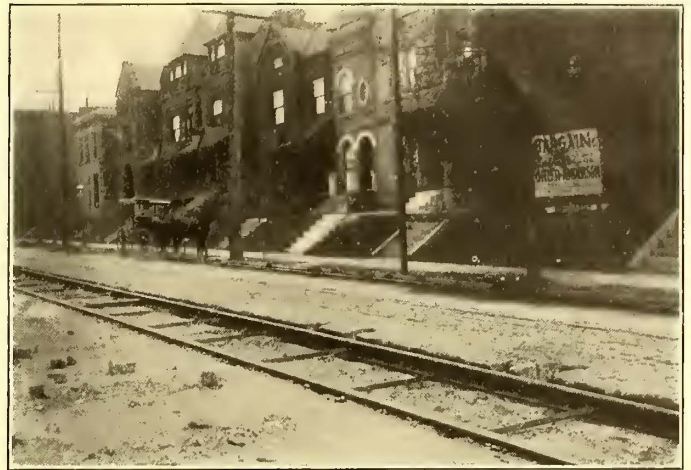
FIG. 7.—VIEW OF TRACK WITH CONDUIT FILLED
