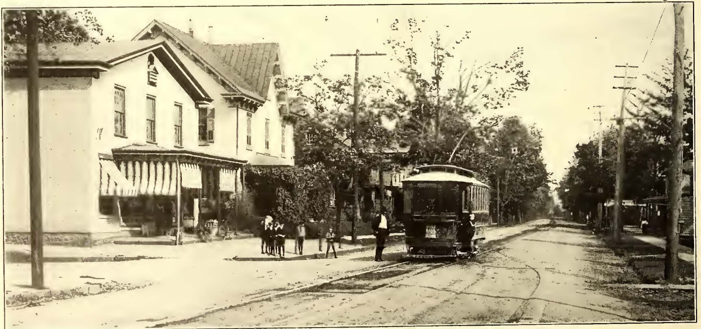
VIEW AT END OF MOORESTOWN LINE, SHOWING SIGN ON SPAN WIRE INDICATING SECTION INSULATOR
