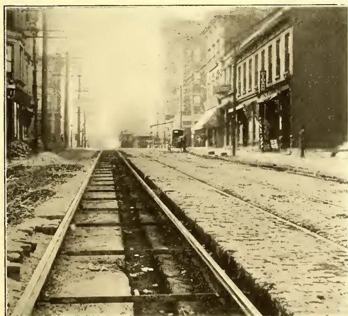
FIG. 8.—VIEW AFTER BORINGS HAVE BEEN RAMMED UNDER RAIL
