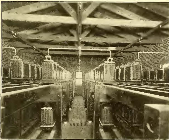
INTERIOR OF WESTMONT BATTERY SUB-STATION
