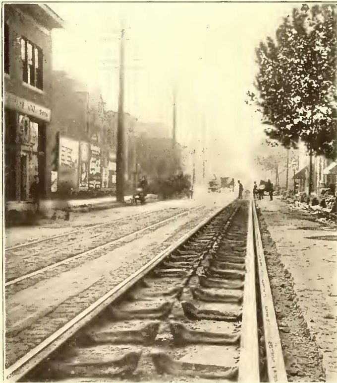
FIG. 4.—VIEW AFTER REMOVAL OF SLOT RAIL
