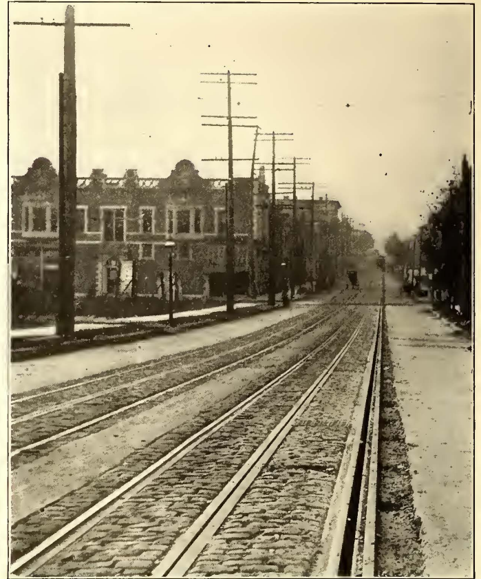
FIG. 3.—VIEW AFTER LAYING OUTSIDE 9-IN. RAIL
