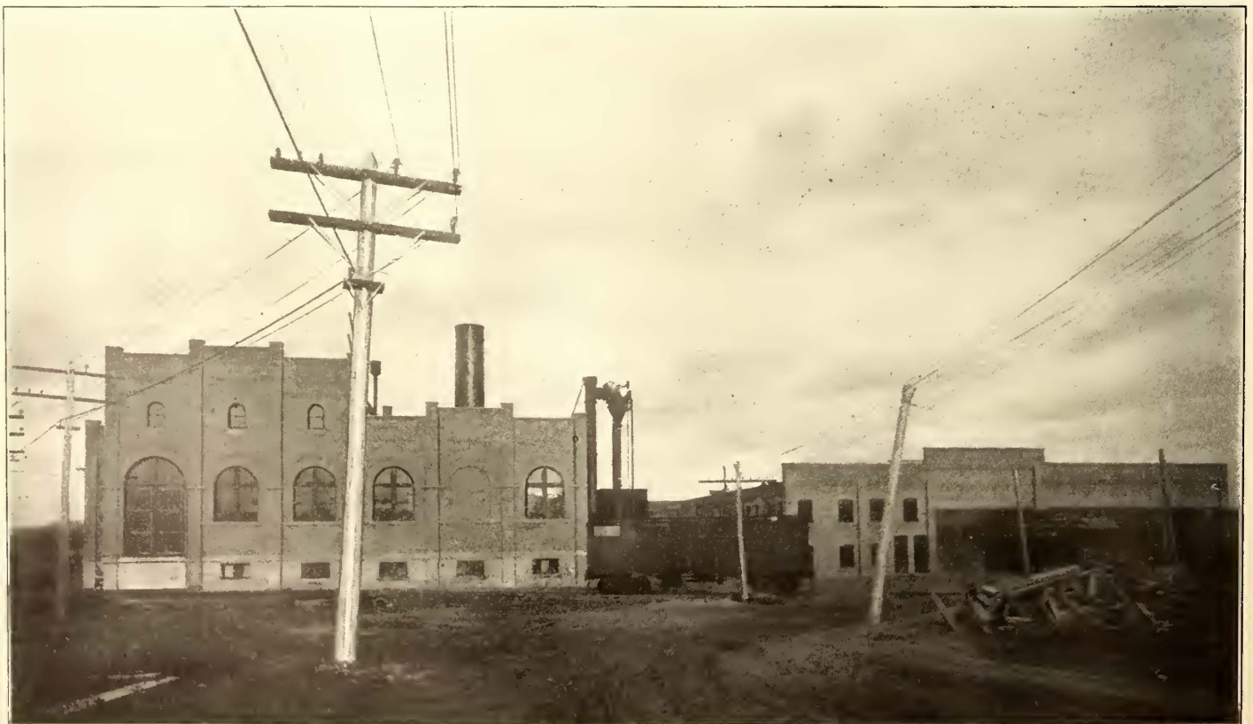
MAIN POWER PLANT, CAR HOUSE AND REPAIR SHOPS
