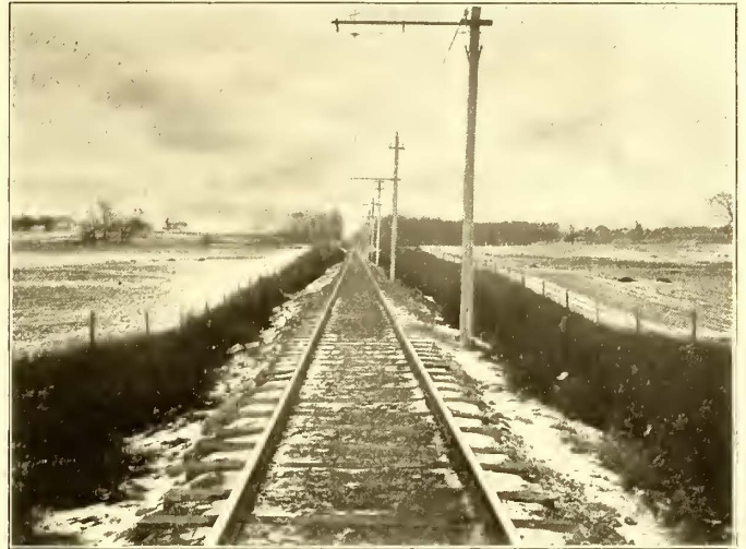
LINE CONSTRUCTION NEAR WOODS
