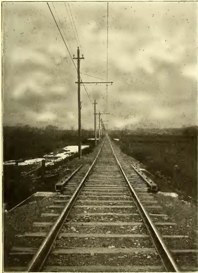
TRACK AND OVERHEAD WORK NEAR VICTOR
