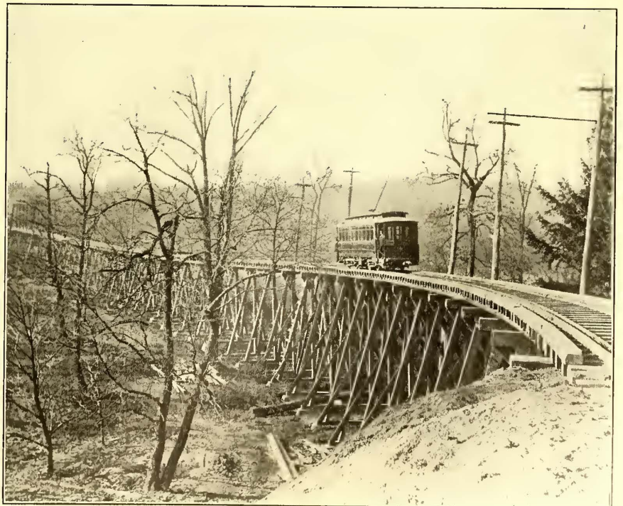
EAST APPROACH TO ELK CREEK TRESTLE
