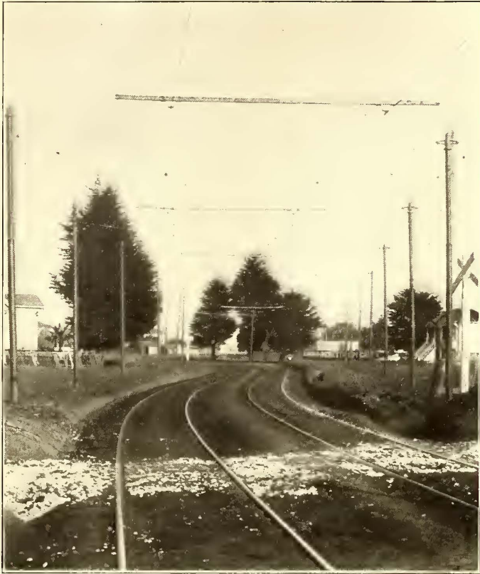
FIG. 17.—DOUBLE-TRACK, SIDE-POLE CONSTRUCTION AT CURVES; WOODEN CROSS-PIECES TO PREVENT DIAMOND TROLLEY FROM TOUCHING SPAN WIRES
