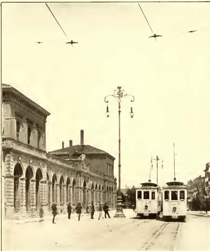
SCENE AT SCHAFFHAUSEN STEAM RAILROAD STATION
