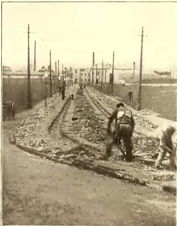
FIG. 3.—LAYING CONTACT SYSTEM IN ABERDEEN
