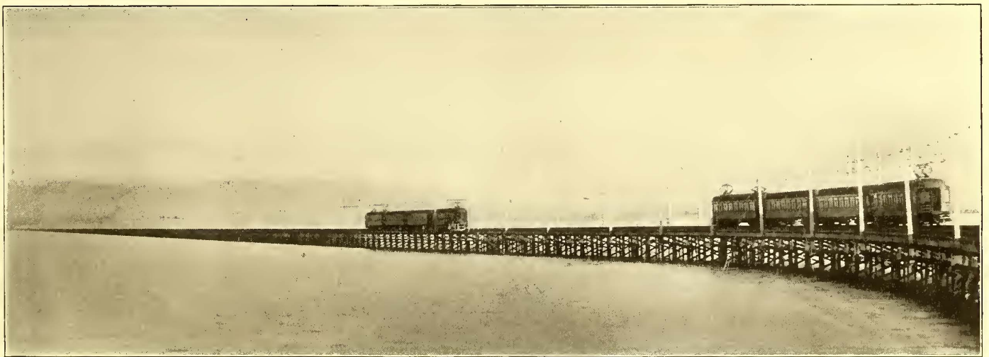
FIG. 10.—VIEW OF PIER LOOKING TOWARD LAND, SHOWING TWO REGULAR 4-CAR TRAINS
