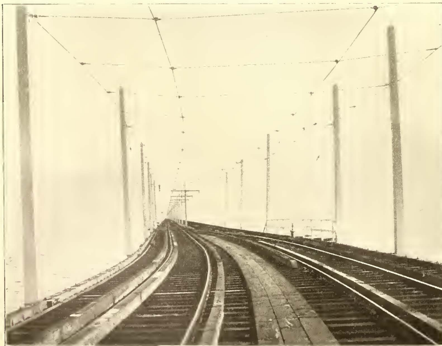
FIG. 9.—SIDE POLE OVERHEAD CONSTRUCTION, WITH CENTER POLE CONSTRUCTION IN DISTANCE ON THE DEPOT-END OF THE PIER
