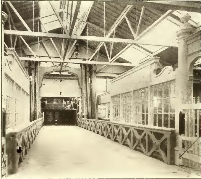
FIG. 7.—HYDRAULICALLY OPERATED APRON, LEADING TO LOWER DECK OF FERRYBOATS AT KEY ROUTE DEPOT; WAITING ROOMS ON BOTH SIDES OF APRON
