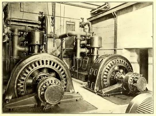
FIG. 6-HIGH-TENSION GENERATING SETS AT LAXEY POWER STATION
