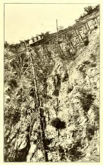
FIG. 6.—LONG BRIDGE ON CABLE INCLINE BETWEEN RUBIO CANYON AND ECHO MOUNTAIN, SHOWING CAR WITH INCLINED SEATS
