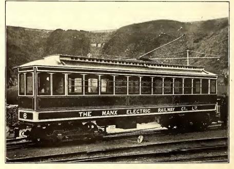
FIG. 19.-MOTOR CAR FOR MANX ELECTRIC RAILWAY
