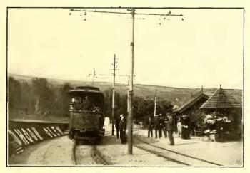
FIG. 16.-TYPICAL OVERHEAD CONSTRUCTION
