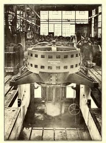
FIG. 2.-VERTICAL MOTOR GENERATOR SET, WITH FRAME
