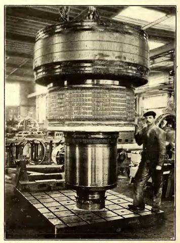
FIG. 3.-VERTICAL MOTOR GENERATOR SET, WITHOUT FRAME
