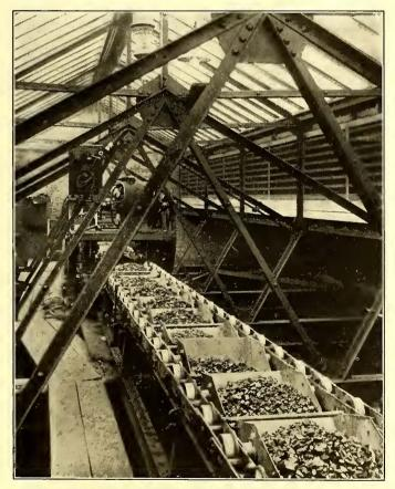
ELECTRICALLY DRIVEN GRAVITY BUCKET CONVEYOR
