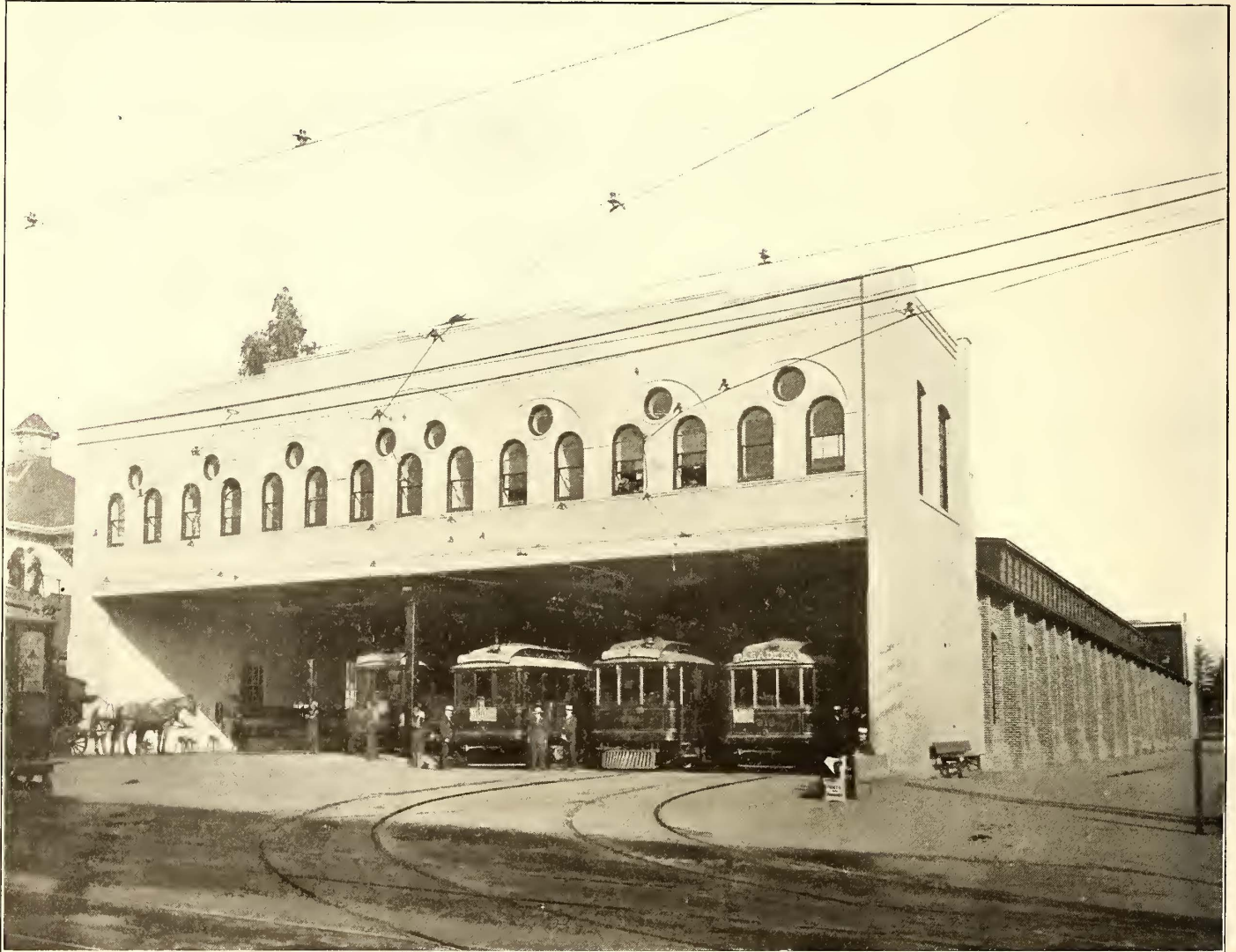
FIG. 27.—PASADENA CAR HOUSE WITH OFFICES ON SECOND FLOOR, SHOWING WEST END FROM WHICH CARS ARE DESPATCHED
