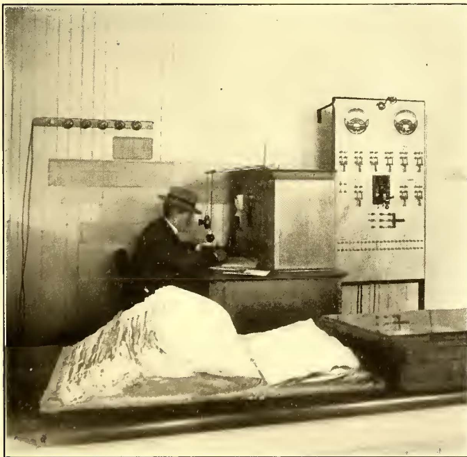
FIG. 29.—DESPATCHER'S DESK IN PASADENA CAR HOUSE
