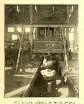
METHOD OF REMOVING ARMATURE
