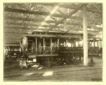
FIG. 19.—PAINT SHOP, SHOWING "A" HORSES USED IN SUPPORTING CAR BODY
