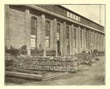
FIG. 13.—SCRAP BIN AND PILES OF WROUGHT-IRON SCRAP READY TO BE FORGED INTO SLABS FOR CAR AXLES
