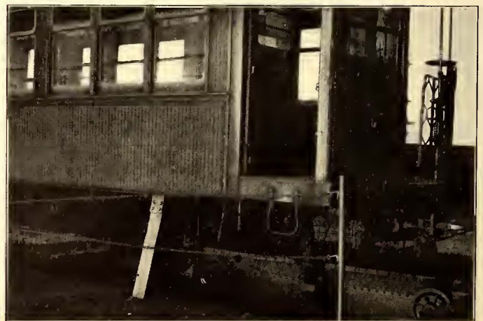
FIG. 4.—CAR SUPPORTED OVER ELEVATOR OPENING, WAITING FOR NEW TRUCK
