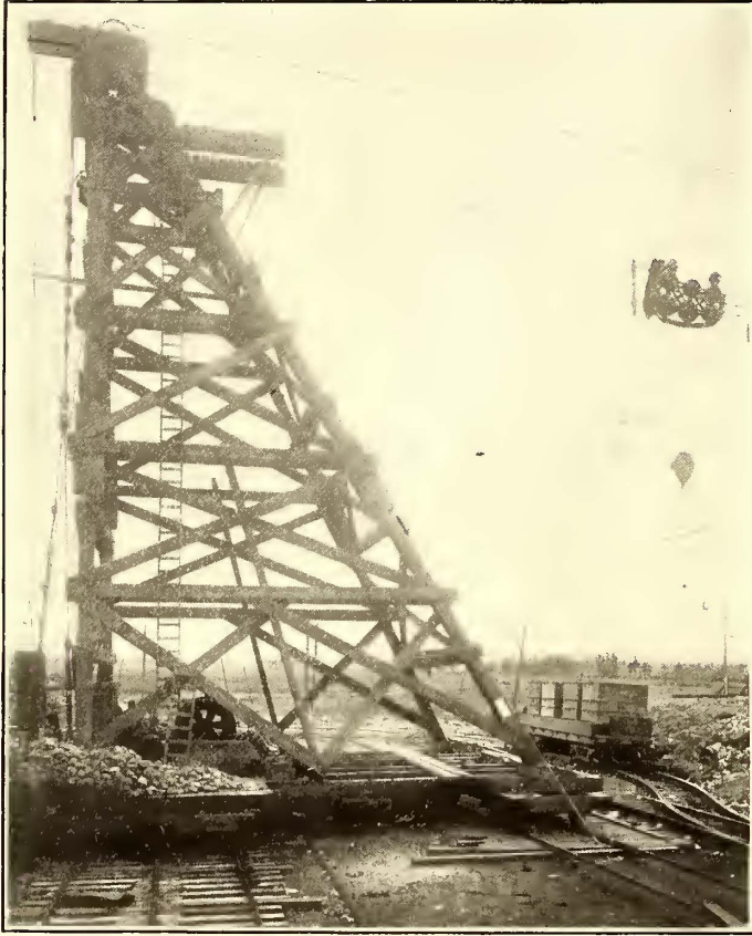
TRAVELING CABLE METHOD OF DUMPING
