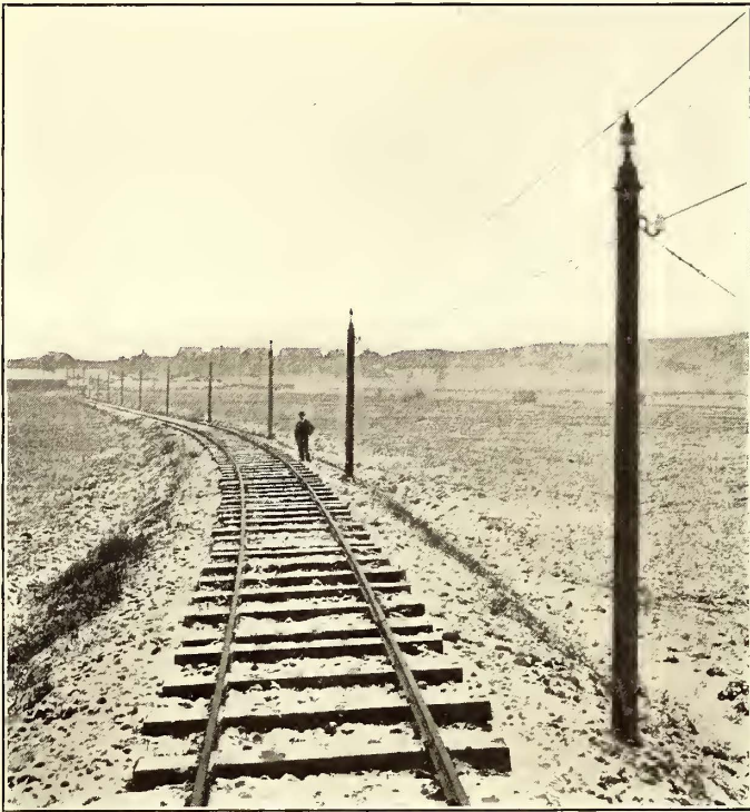
FIG. 13.—VIEW OF AERIAL CONSTRUCTION OF SINGLE-PHASE RAILWAY
