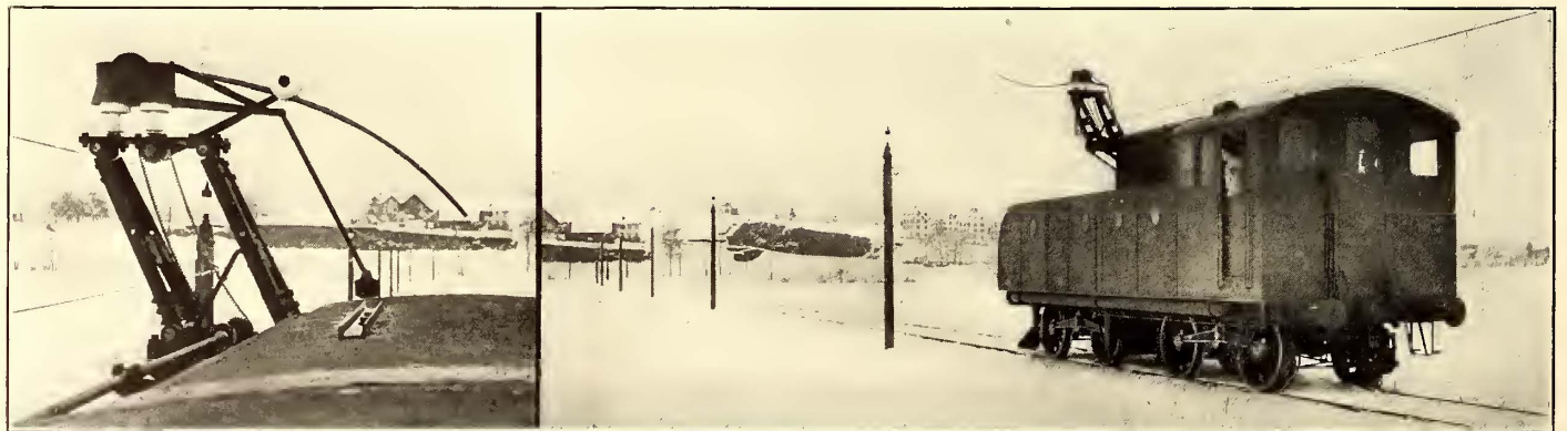
FIGS. 14 AND 15.—FLEXIBLE-ROD CURRENT COLLECTOR IN USE ON EXPERIMENTAL LINE
