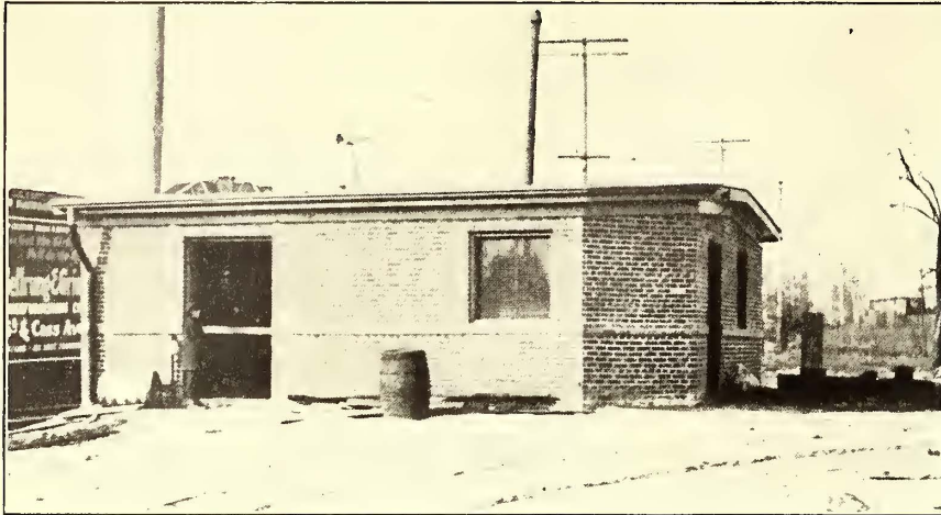
COMPRESSING STATION AT DE HODIAMONT—CAPACITY, THREE COMPRESSORS
