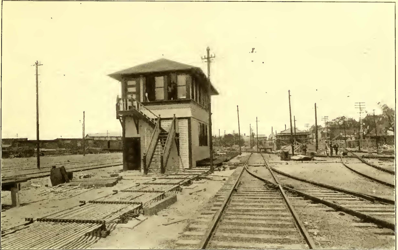
FIG. 6.—LOOKING NORTH FROM THE ELEVATED TRAIN TERMINAL TRACKS, SHOWING CENTRAL SWITCH AND SIGNAL TOWER AND THE OPERATING PIPE LINES
