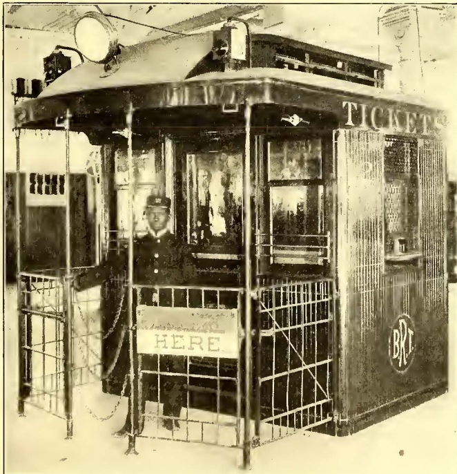
FIG. 4.—DETAIL VIEW OF THE NOVEL TICKET BOOTH
