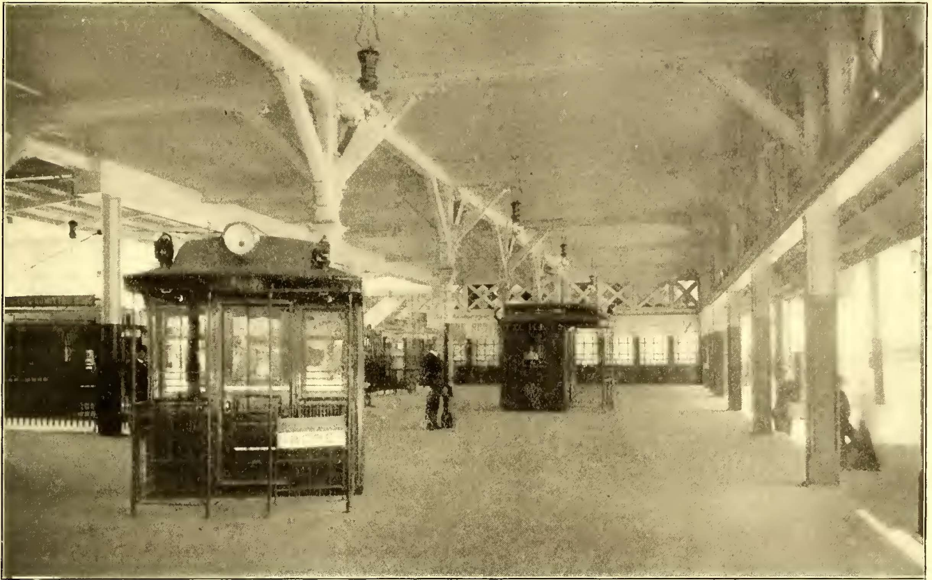
FIG. 3.—THE ELEVATED TERMINAL DEPOT, SHOWING USE OF AN UNUSUAL FORM OF TICKET BOOTH, RESEMBLING THE END OF AN ELEVATED CAR
