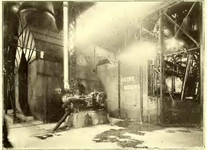
HEINE SAFETY BOILERS IN POWER PLANT
