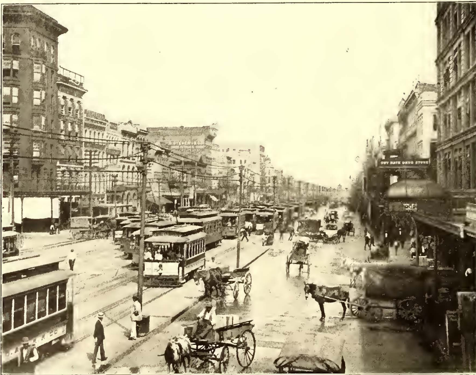
VIEW ON CANAL STREET, SHOWING FIVE LINES OF TRACK
