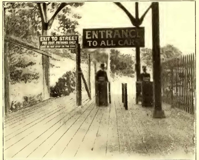
EXIT TO DEPARTURE PLATFORM FOR CARS LEAVING PARK, AND PASSAGE TO STREET
