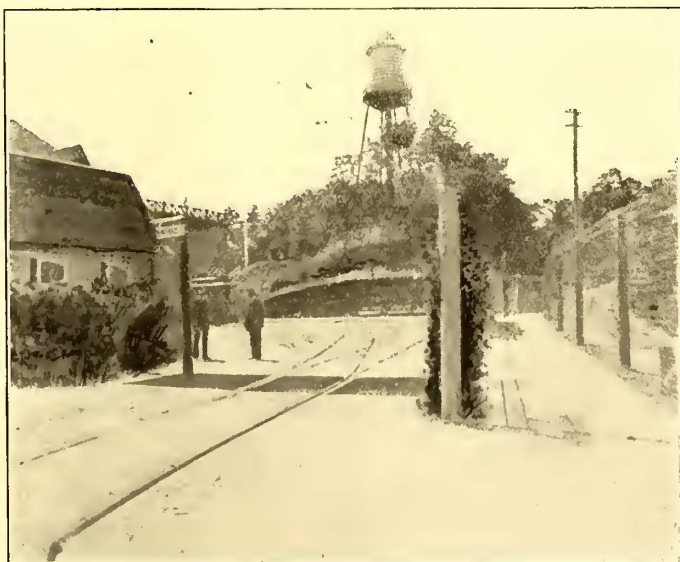
OPENING TO STREET FROM THE CAR TERMINAL, SHOWING PIT TO PREVENT ENTRANCES AT THAT POINT
