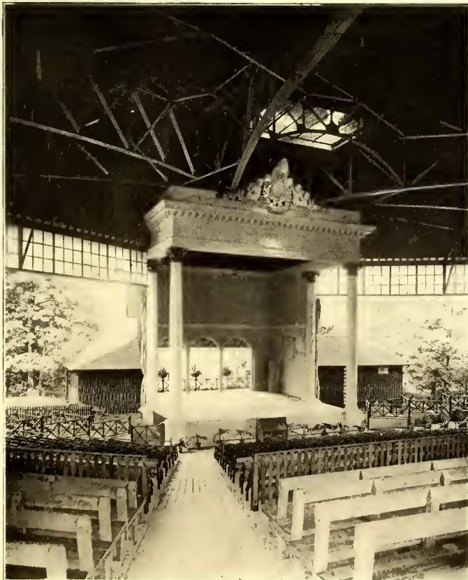
INTERIOR VIEW OF THEATER, SHOWING NEW STAGE
