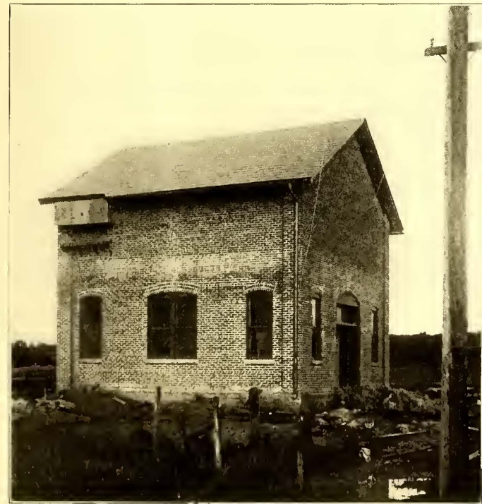
SUB-STATION ON THE SPRINGFIELD, TROY & PIQUA RAILWAY
