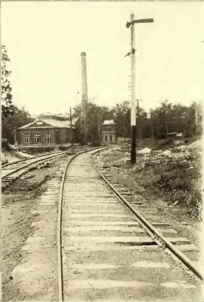
INTERLOCKER AT ERIE CROSSING, WITH POWER HOUSE IN THE BACKGROUND
