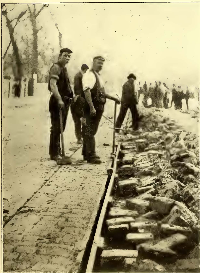
BREAKING UP OLD TRACK WITH SLEDGE HAMMERS AND WEDGES IN LONDON
