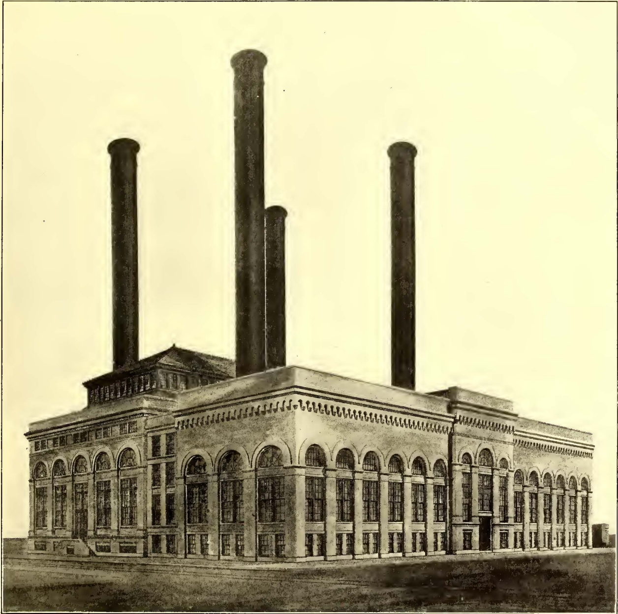
PERSPECTIVE VIEW OF NEW POWER STATION, NOW BEING ERECTED IN NEW ORLEANS
