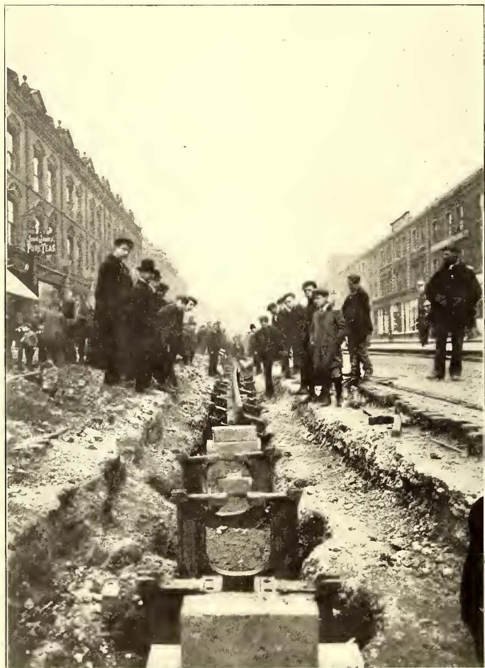
TRENCH WITH YOKES IN AND SLOT RAIL
