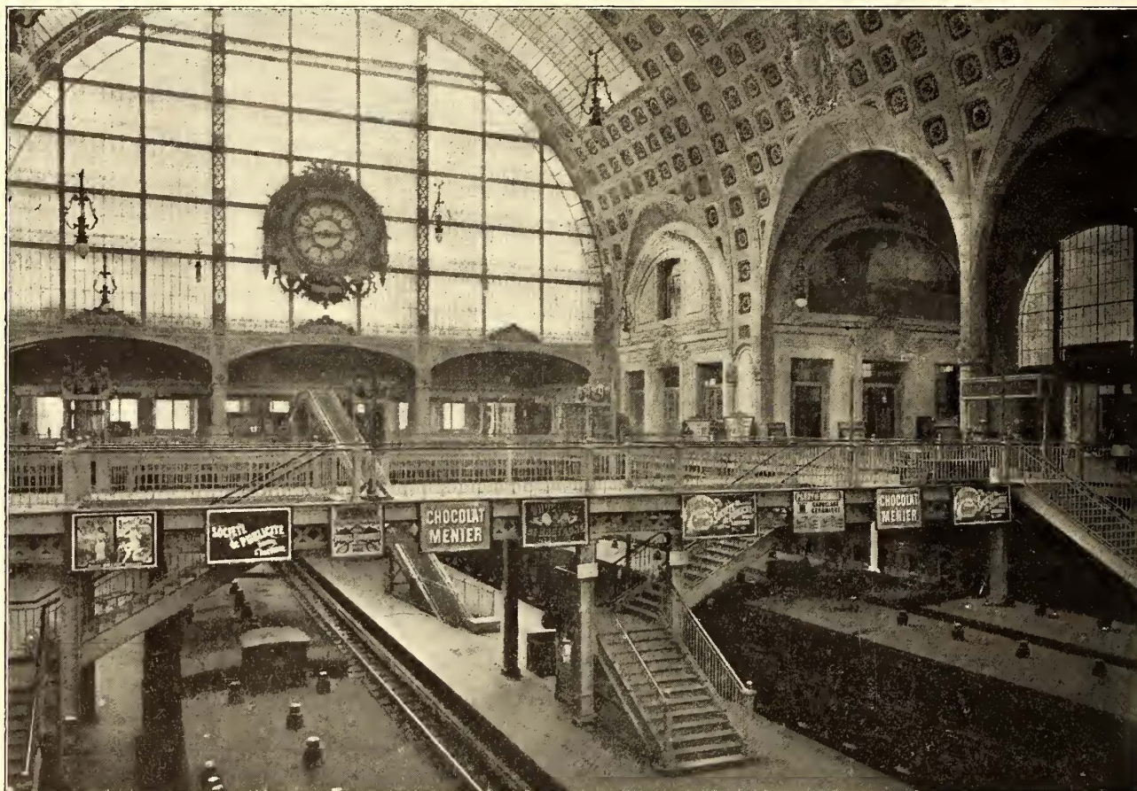
INTERIOR OF ORSAY RAILROAD STATION, THE TERMINUS OF THE ELECTRIC SERVICE—THE ELECTRIC ELEVATOR FOR HOISTING TRUNKS AND OTHER BAGGAGE IS SHOWN AT THE REAR OF THE MIDDLE PLATFORM
