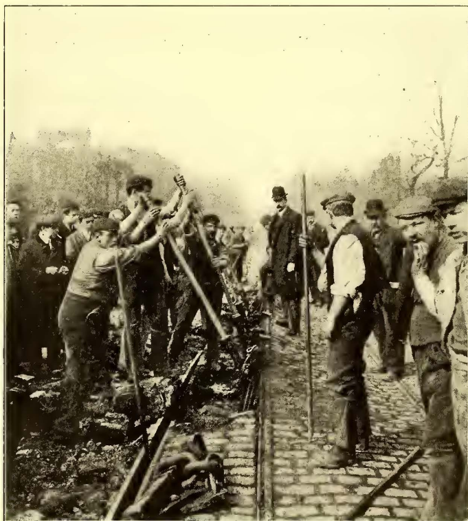
JACKING UP OLD TRACK—RAIL LIFTER IN FOREGROUND
