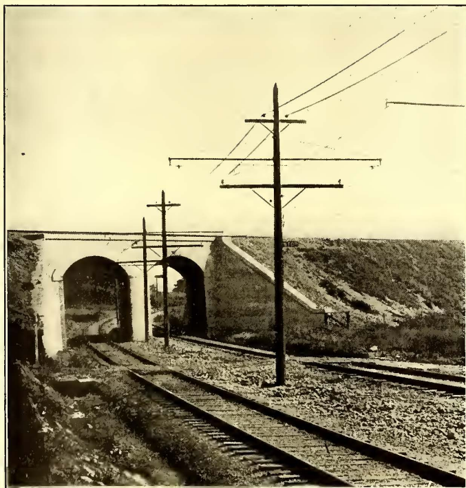
UNDER CROSSING OF BALLSTON LINE WITH BOSTON & MAINE CULVERT, SHOWING ALTERNATING AND DIRECT-CURRENT TROLLEY WIRES
