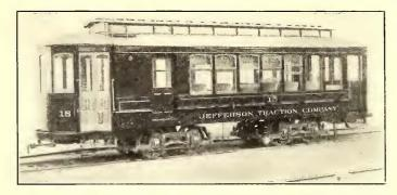
COMBINED SEMI-CONVERTIBLE AND BAGGAGE CAR FOR THE JEFFERSON TRACTION COMPANY
