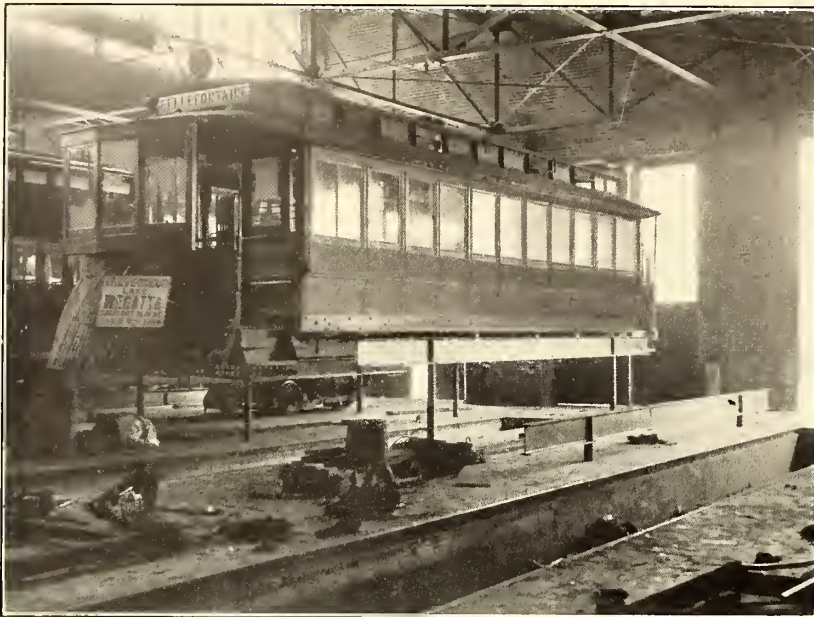
CAR HOISTS IN ST. LOUIS TRANSIT COMPANY'S SHOPS
