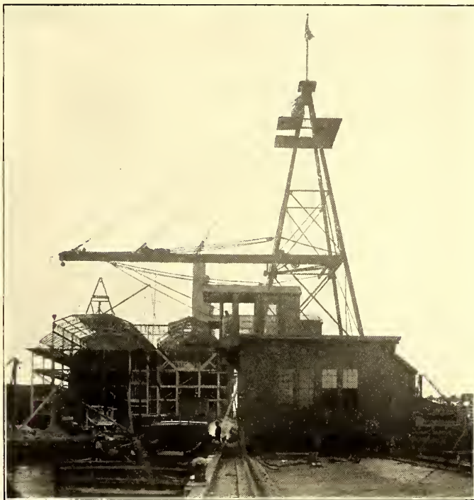
THE TRAVELING HOISTING TOWER UPON THE COAL UNLOADING PIER, FOR HANDLING COAL TO THE CONVEYOR SYSTEM
