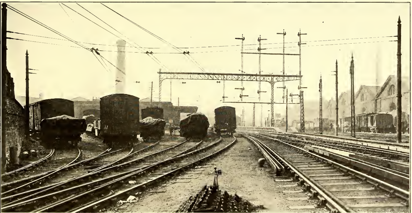
A VIEW OF THE FREIGHT YARD AT NEWCASTLE, SHOWING OVERHEAD WIRES AND THIRD RAIL
