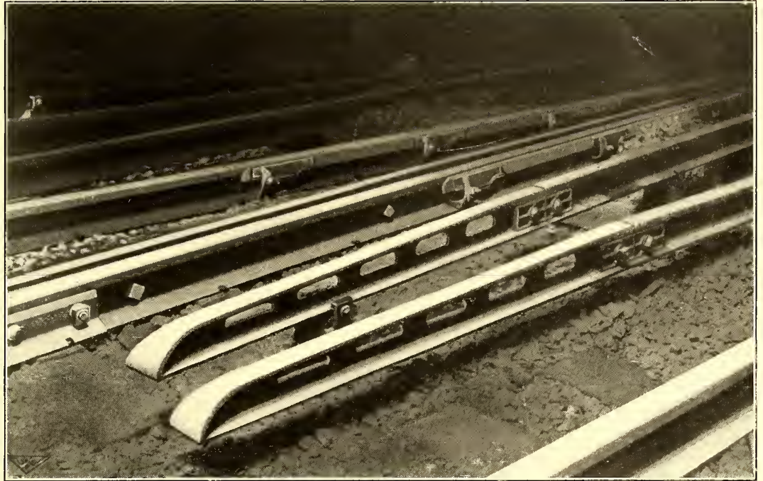
VIEW OF RUNNING AND CONTACT RAILS IN THE TUNNEL, SHOWING SPECIAL TYPE OF END INCLINE USED UPON CONTACT RAILS
