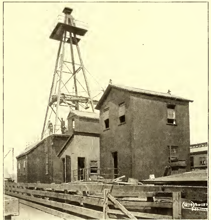
THE TRAVELING HOISTING TOWER UPON THE COAL UNLOADING PIER, FOR HANDLING COAL TO THE CONVEYOR SYSTEM
