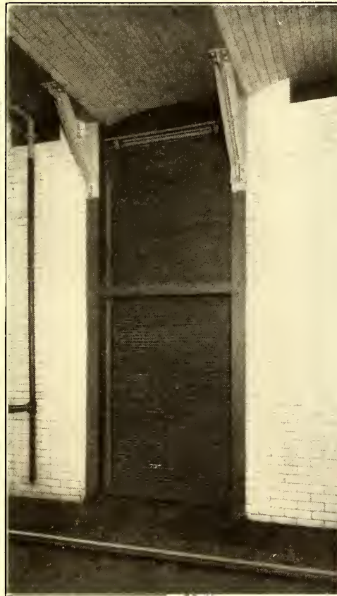
VIEWS OF THE CABLE MANHOLES IN THE SIDE WALL OF THE TUNNEL, SHOWING ROLLING SHUTTER DOORS FOR READY ACCESS
