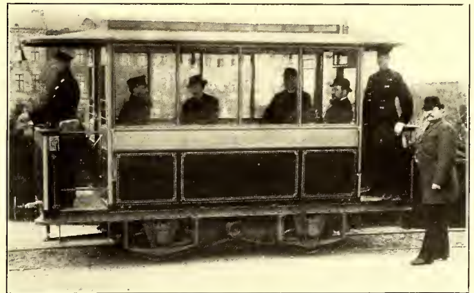
CAR USED IN 1881 ON THE GROSS-LICHTERFELDE LINE, TAKING CURRENT FROM ONE RAIL AND USING THE OTHER FOR THE RETURN CIRCUIT
