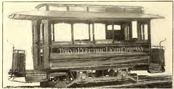
HORSE CAR TRANSFORMED FOR ELECTRIC SERVICE
