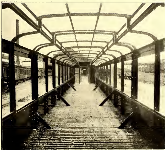
Side Plates and Corrugated Flooring in Place
