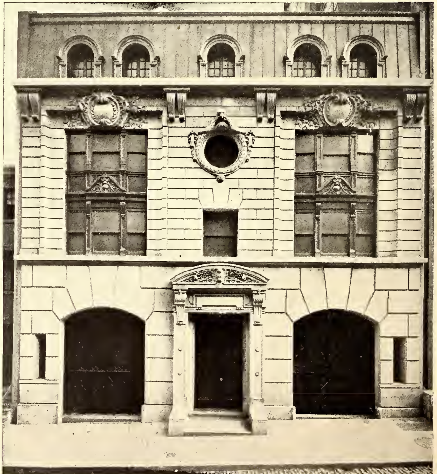
EXTERIOR VIEW OF SUB-STATION NO. 11, SHOWING ARTISTIC ARCHITECTURAL TREATMENT
