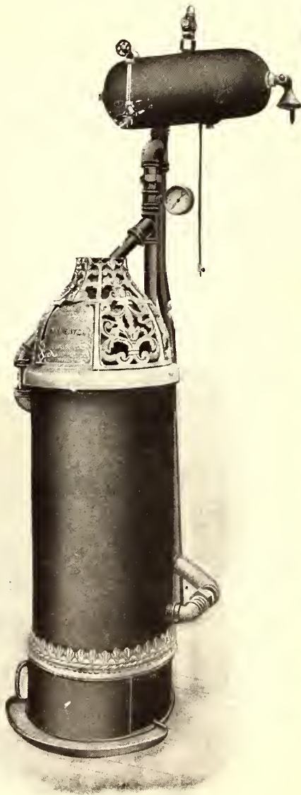
HOT-WATER CAR HEATER COMPLETE
