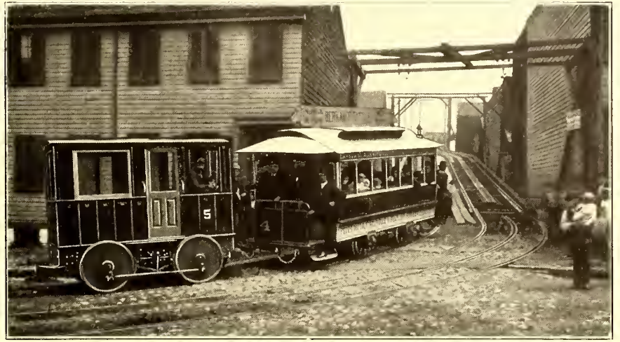
FIG. 11.—MOTOR TRAIN CHANGING FROM TROLLEY TO CONDUIT—PITTSBURG, 1887-8
