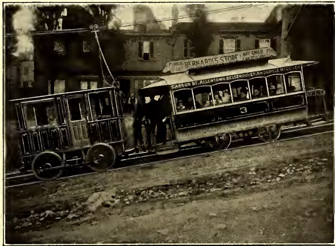
FIG. 10.—MOTOR TRAIN ON 15 PER CENT GRADIENT—PITTSBURG, 1887-8
