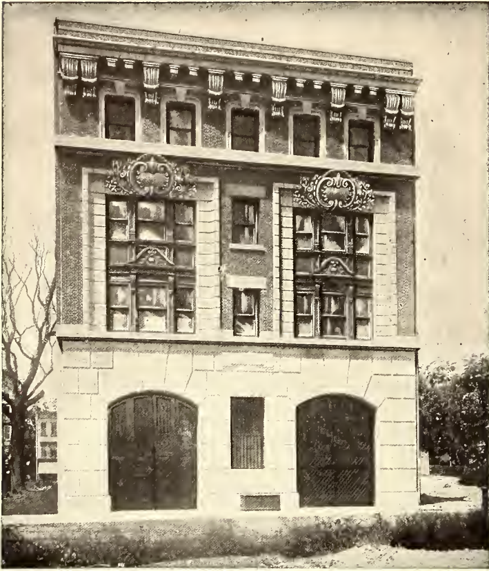
EXTERIOR OF SUB-STATION NO. 18
