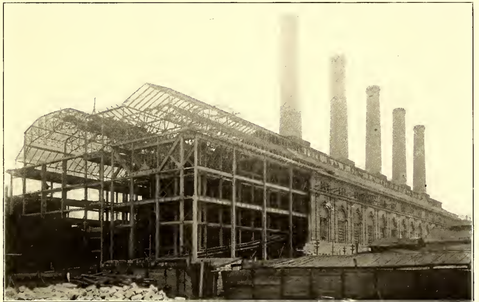
EXTERIOR VIEW OF THE POWER PLANT DURING CONSTRUCTION, SHOWING STEEL WORK
