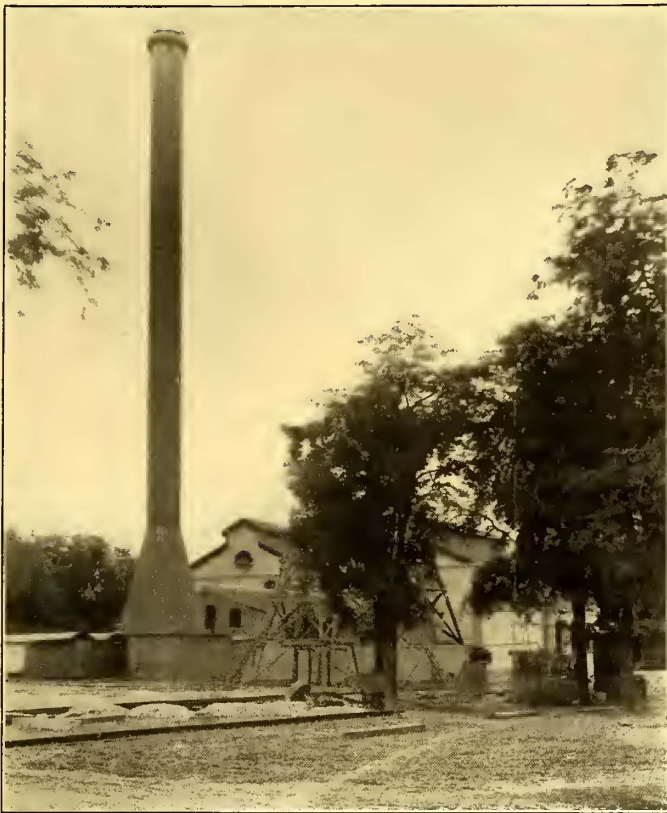
MANDALAY POWER HOUSE AND CHIMNEY
