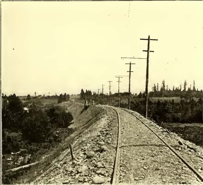
FIG. 9.—HEAVY FILL ACROSS JOHNSON CREEK VALLEY 35 FT. TO 50 FT. HIGH AND 3200 FT. LONG
