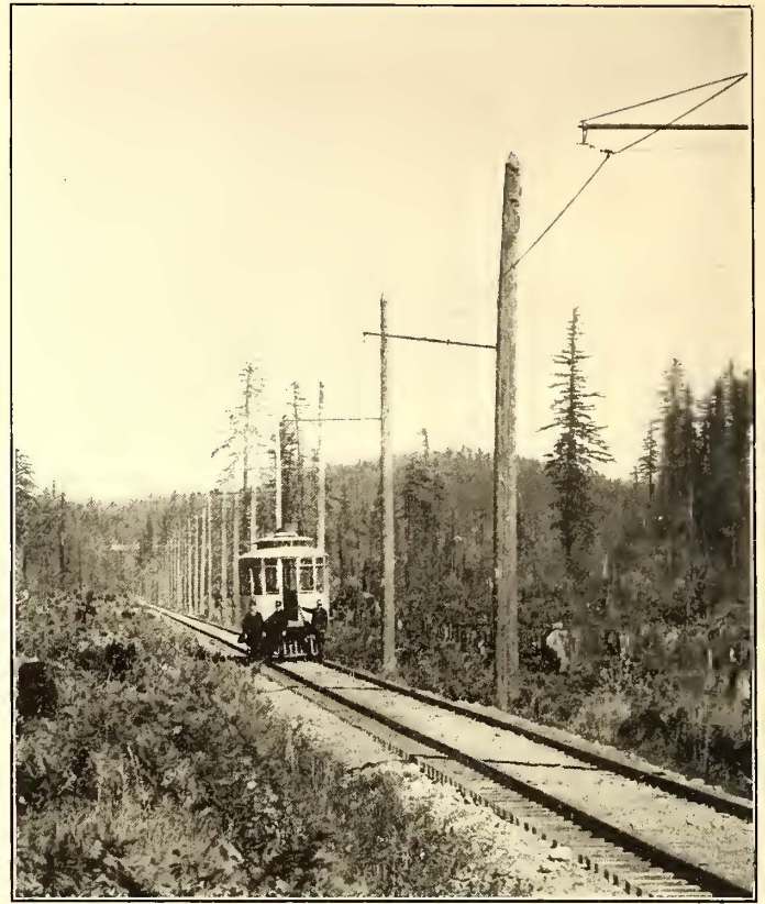
FIG. 7.—VIEW ON CAZADERO LINE, SHOWING STANDARD TRACK
