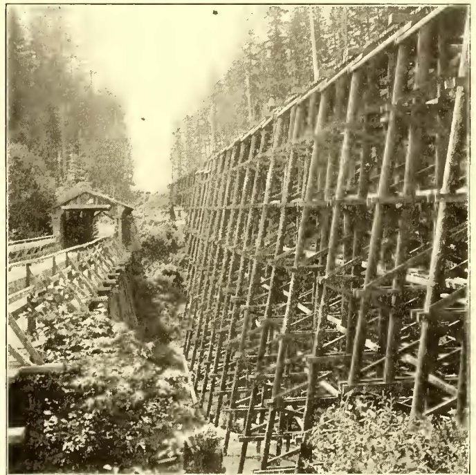
FIG. 14.—EAGLE CREEK PILE TRESTLE, 95 FT. HIGH (OLD COUNTRY ROAD BRIDGE AT LEFT)
