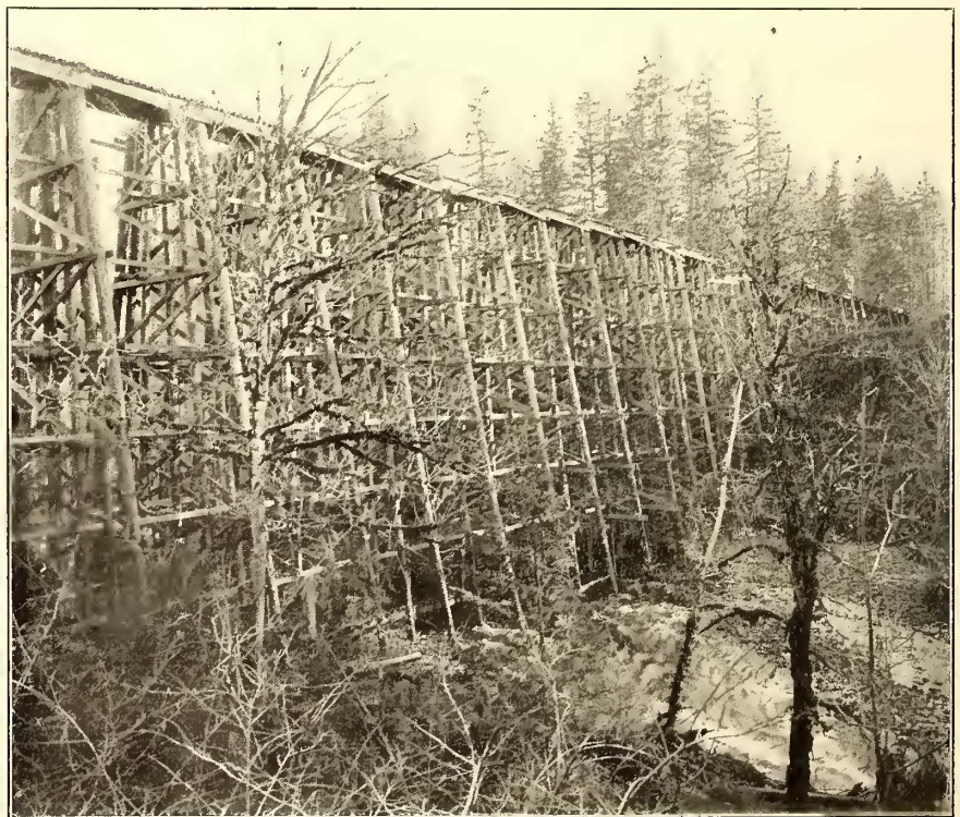
FIG. 15.—EAGLE CREEK 95-FT. PILE TRESTLE
