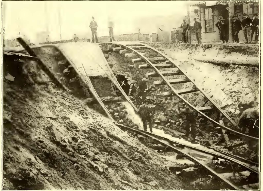
WASHOUT AT THE TERMINAL OF THE FILLMORE STREET LINE OF THE UNITED RAILROADS OF SAN FRANCISCO. THE X SHOWS THE OPENING OF THE MAIN SEWER WHICH CAVED IN
