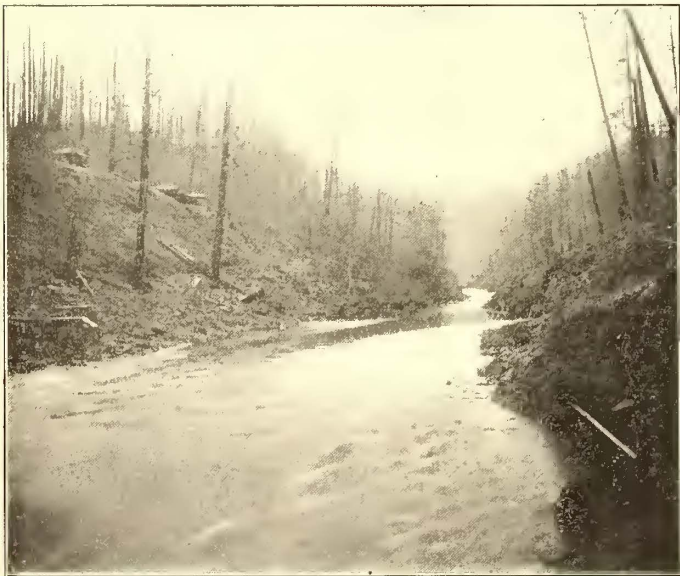
FIG. 23.—SITE OF DAM ON CLACKAMAS RIVER AT CAZADERO WHERE 25,000 HP IS TO BE DEVELOPED
