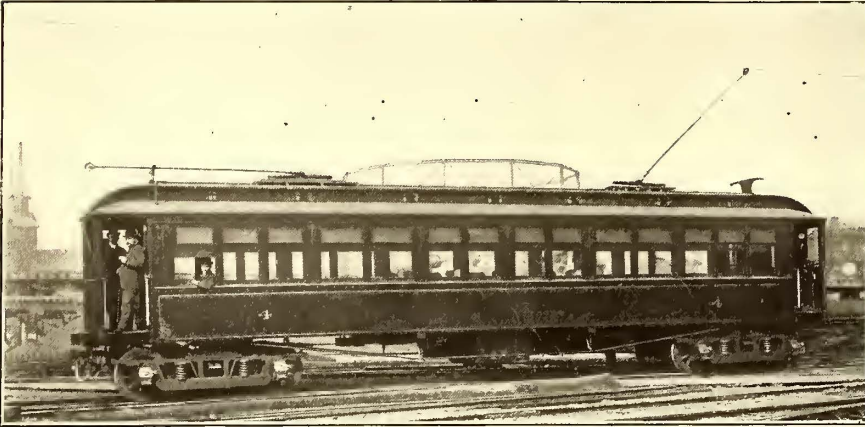
FIG. 1.—CAR ON THE INTER-WORKS RAILWAY EQUIPPED WITH A. C. APPARATUS. TROLLEY AND LINE CONSTRUCTION FOR 1000 VOLTS AND LESS
