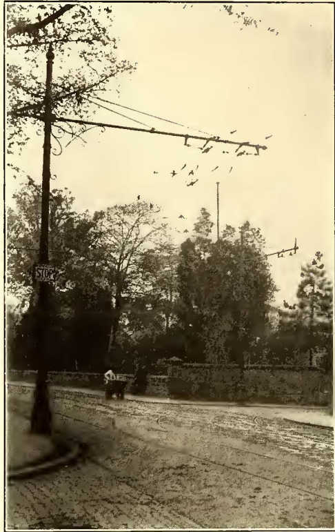
BRACKET-ARM CONSTRUCTION AT OSMASTON ROAD
