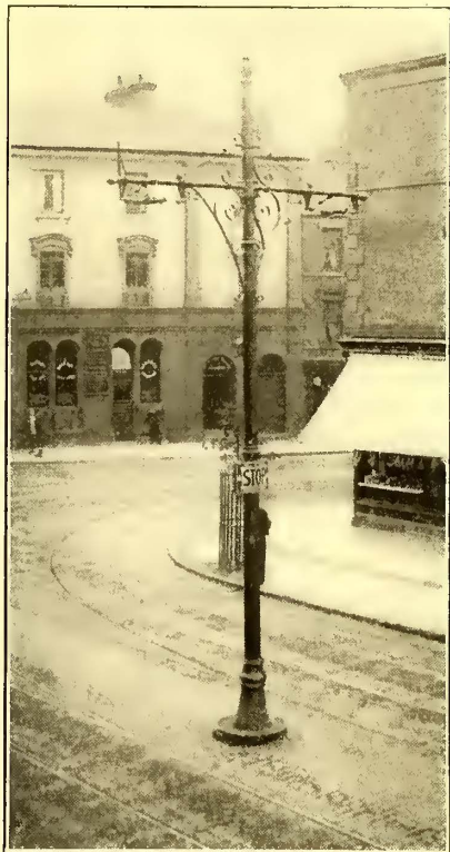
CENTER-POLE CONSTRUCTION ON LONDON ROAD, DERBY
